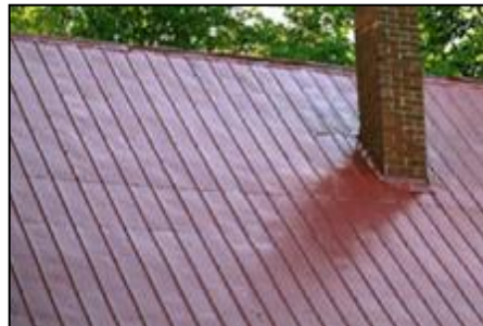
Standing Seam Metal Roof
