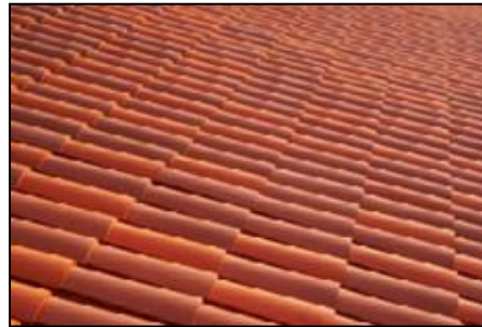
Clay Tile Roof
