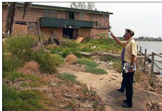
Figure 7-3: Screening the exterior of a damaged structure
