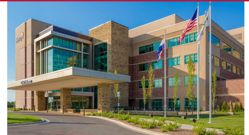
Rebuilt Mercy Hospital as it looks today
