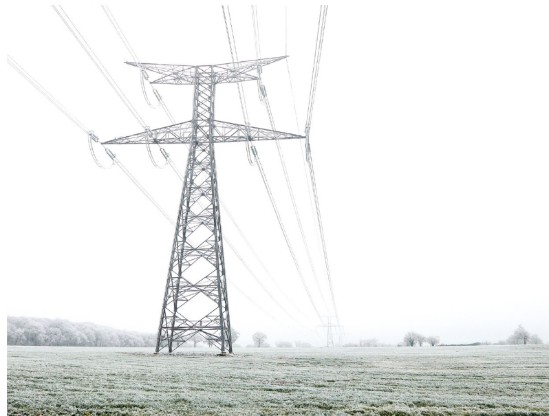
Ice covers electrical sources
