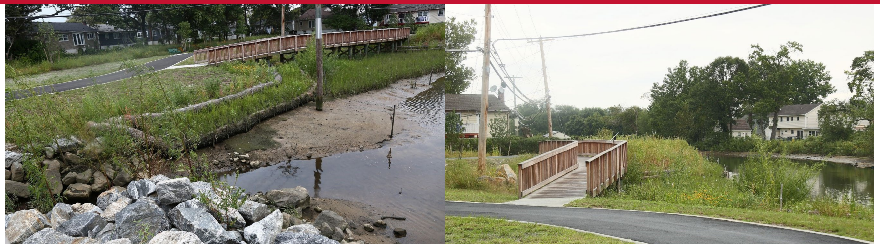
Natural coastal buffer designed to reduce erosion and sedimentation and improve wildlife habitat
