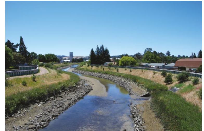
Northern California Flood Control Mitigation Source: FEMA. Loss Avoidance Study: Northern California Flood Control Mitigation
