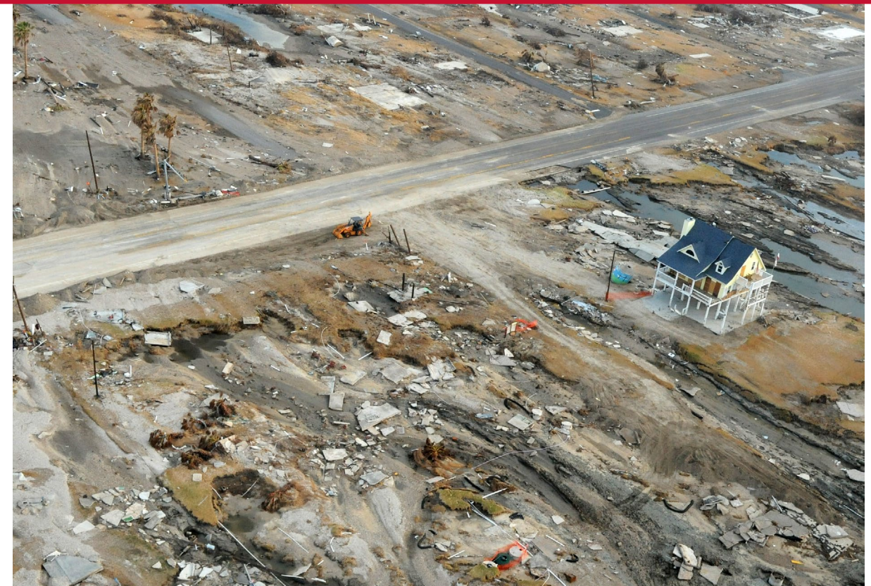
Hurricane destruction surrounding a standing house Source: Jocelyn Augusitno/FEMA / Public domain, https://upload.wikimedia.org/wikipedia/commons/5/55/Hurricane_Ike_Gilchrist_damage_edit.jpg
