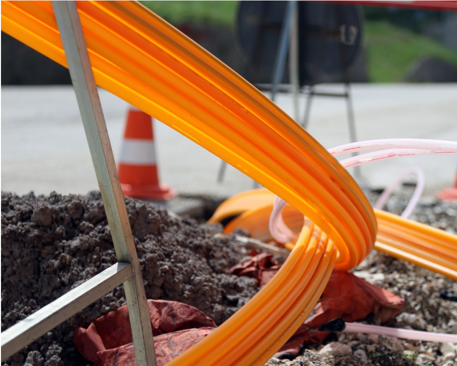
Excavation for the laying of optical fiber Source: Shutterstock
