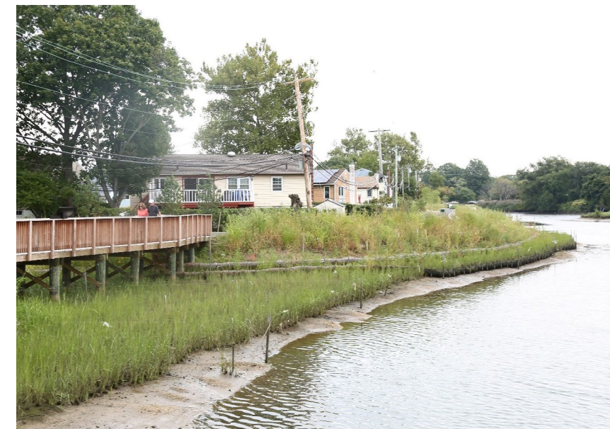
Natural coastal buffer designed to reduce erosion and sedimentation and improve wildlife habitat
