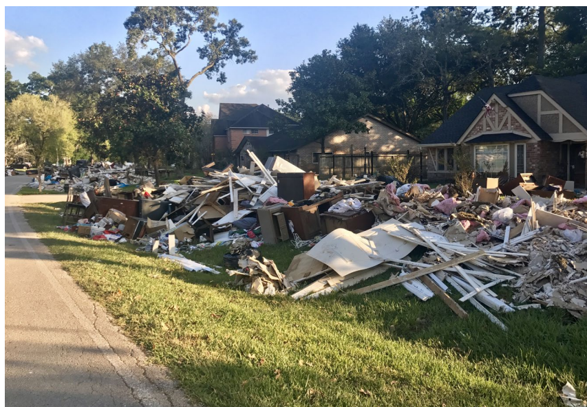
Hurricane Harvey flood damage to homes in Harris County, TX
