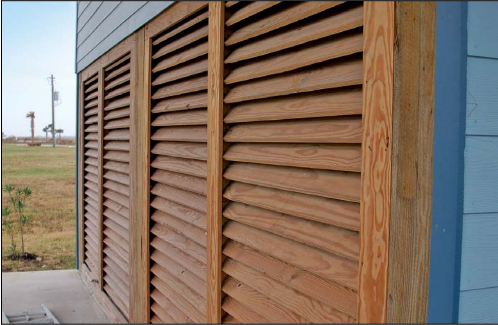
Figure 5: Compliant, fixed, wood louvers installed between pilings
