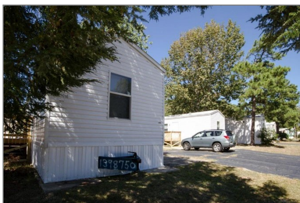
One of several MHUs provided by FEMA in Crestwood, New Jersey following Hurricane Sandy.
