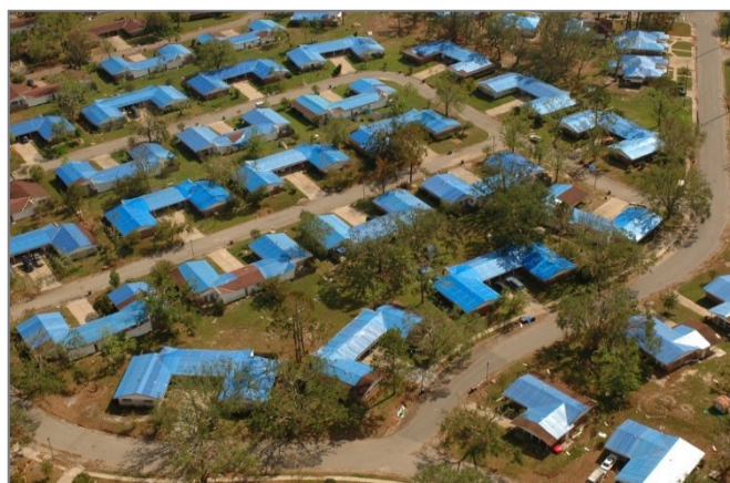
US Army Corps of Engineers' Blue Roof Program helps to prevent further damage to structures as a result of Hurricane Katrina in Biloxi, Mississippi.
