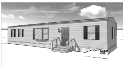
Mobile home with skirting
