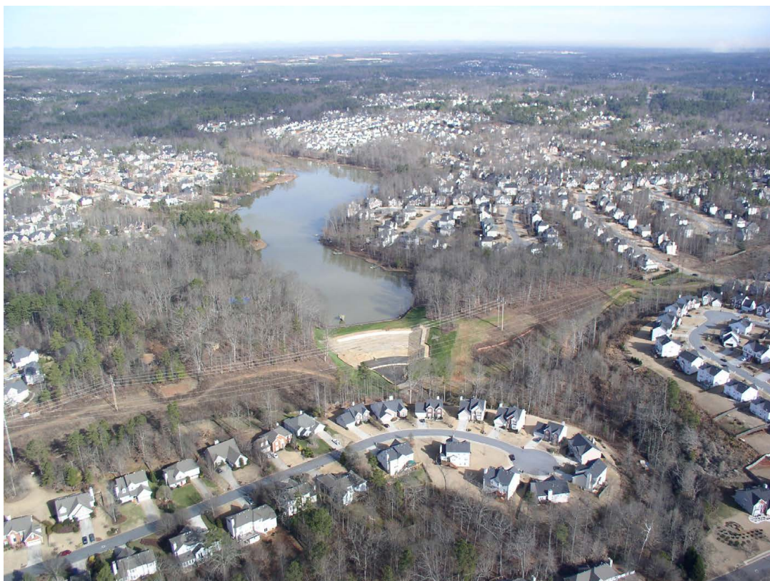
Figure 2.3.2. This dam is considered high hazard potential because its failure would impact the community directly downstream and could result in loss of life and property. (Source: NRCS, 2014)
