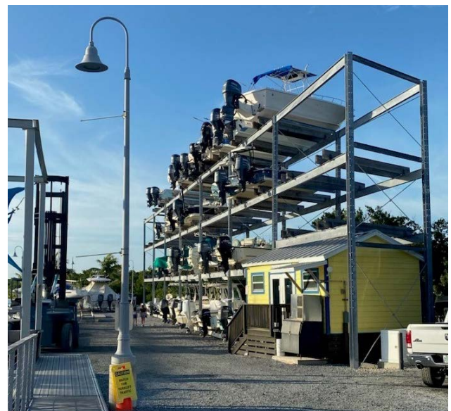
Figure 5.5.7. An example of an outdoor dry-stack storage facility (Source: Brendan McGinley, 2021).
