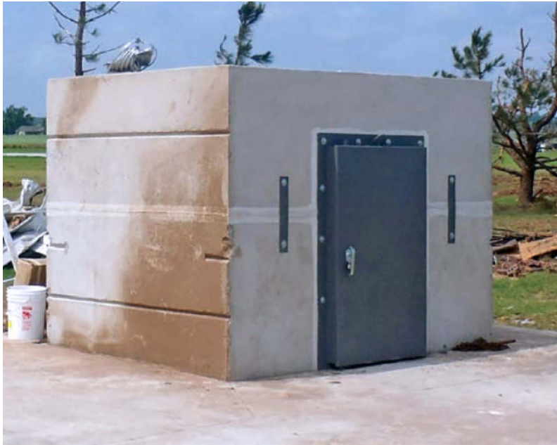
Figure 4.3.18. Data collection gateways should be protected against wind by placing them in storm shelters.
