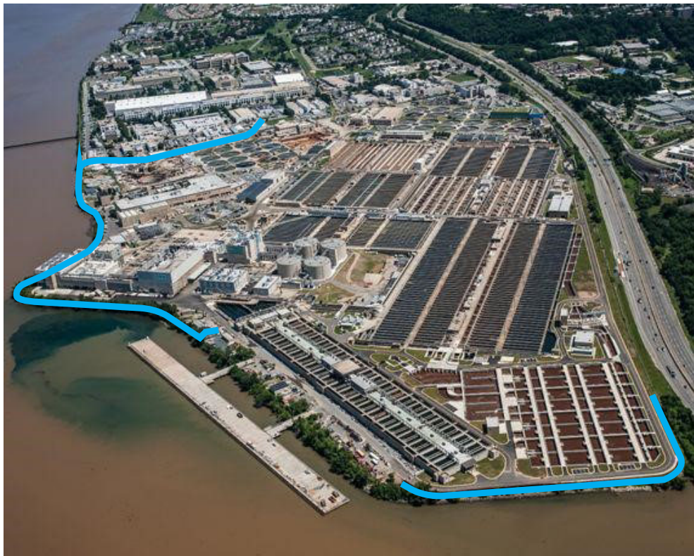
Figure 4.2.2. Constructing a flood wall that extends above the 500-year flood elevation can help protect a wastewater treatment plant from flood damage. The blue lines indicate the approximate location of the planned floodwall for this treatment facility. (U.S. Environmental Protection Agency [EPA], 2021)
