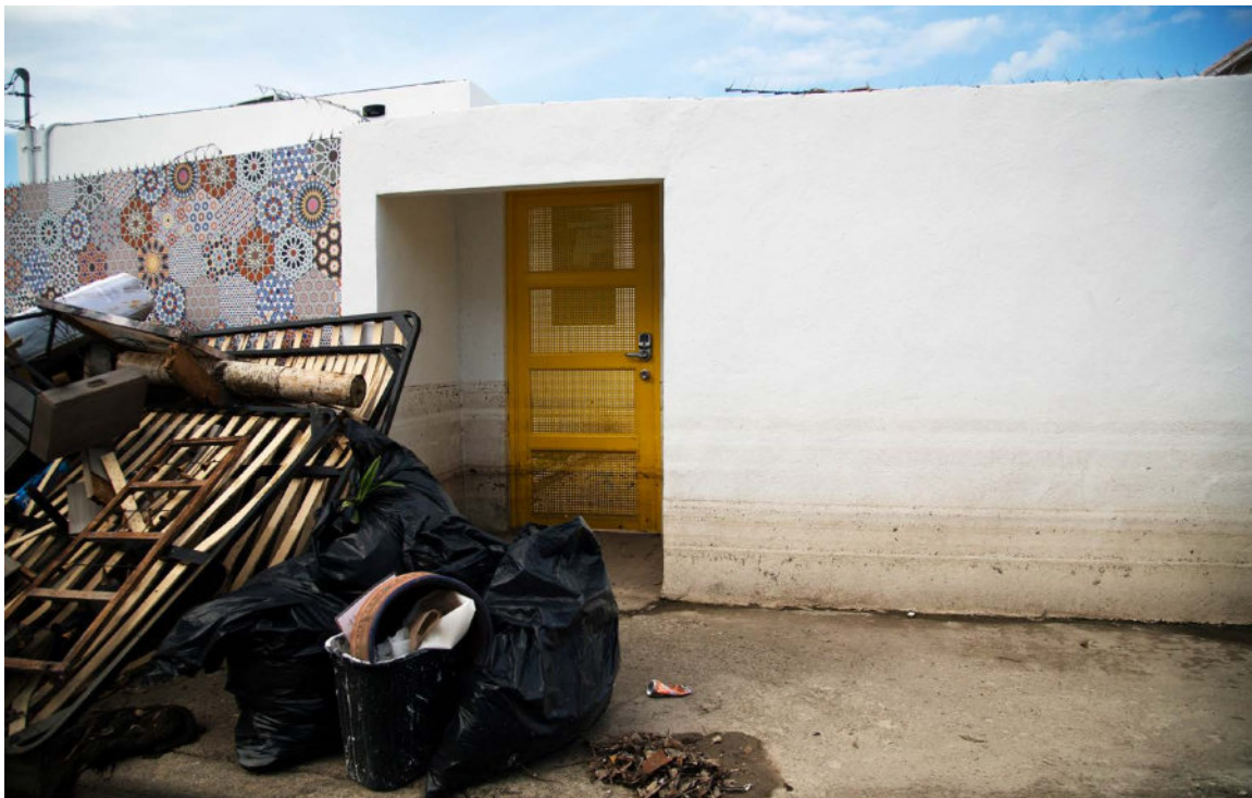
Figure 0.0.1. Measuring high-water marks can help establish flood depth.
