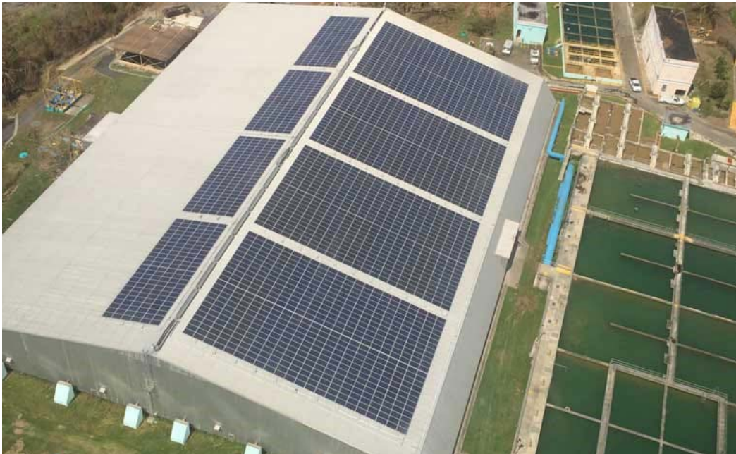
Figure 4.2.5. Installing renewable energy resources like solar panels can provide a standby source of power for wastewater treatment facilities. (National Renewable Energy Laboratory [NREL], 2017)
