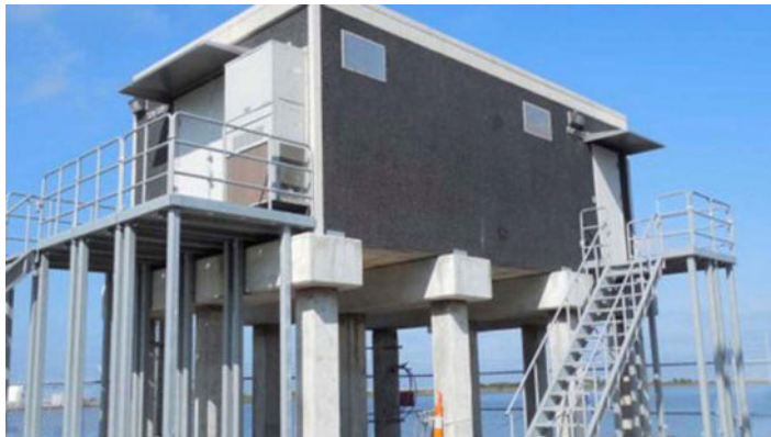
Figure 4.3.9. Elevating a control house in coastal areas can protect it against damage from storm surge and flooding. (Source: Modular Connections, 2020)
