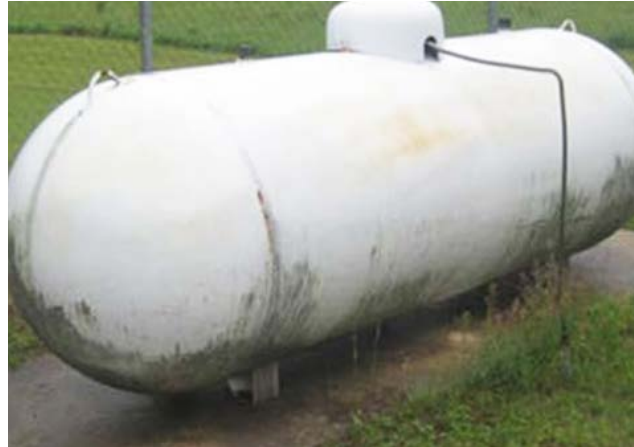
Figure 4.1.5. Secure tanks with non-corrosive straps to prevent flotation. (Source: U.S. Environmental Protection Agency [EPA], 2014)
