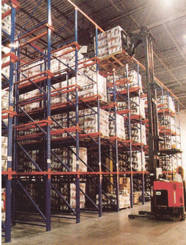
Figure 10-6 Seismic design criteria for steel storage racks of the type used in large warehouses and big-box retail stores are included in the building code.
