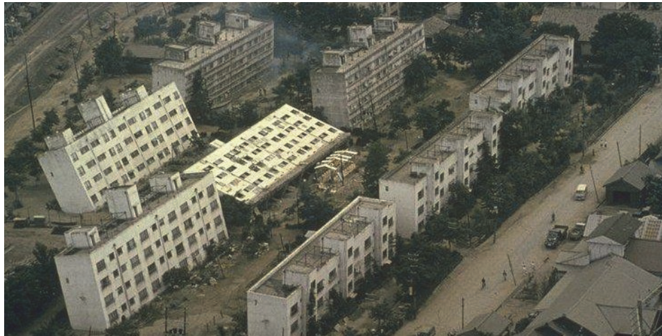
Figure 1-11 Liquefaction-induced settlement of apartment buildings in the 1964 Niigata Earthquake in Japan (from University of Washington).
