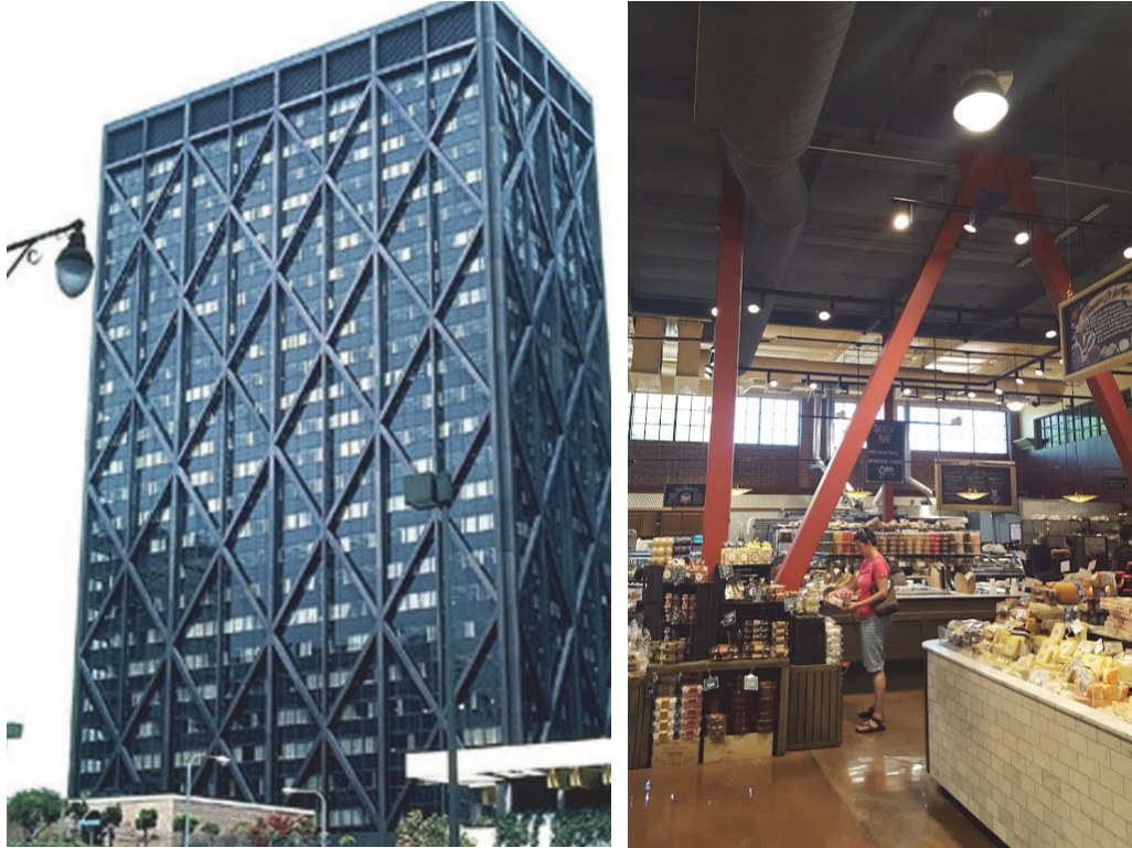
Figure 5-8 Steel braced frames left exposed on the exterior of a high-rise (left) and inside a grocery store (right).
