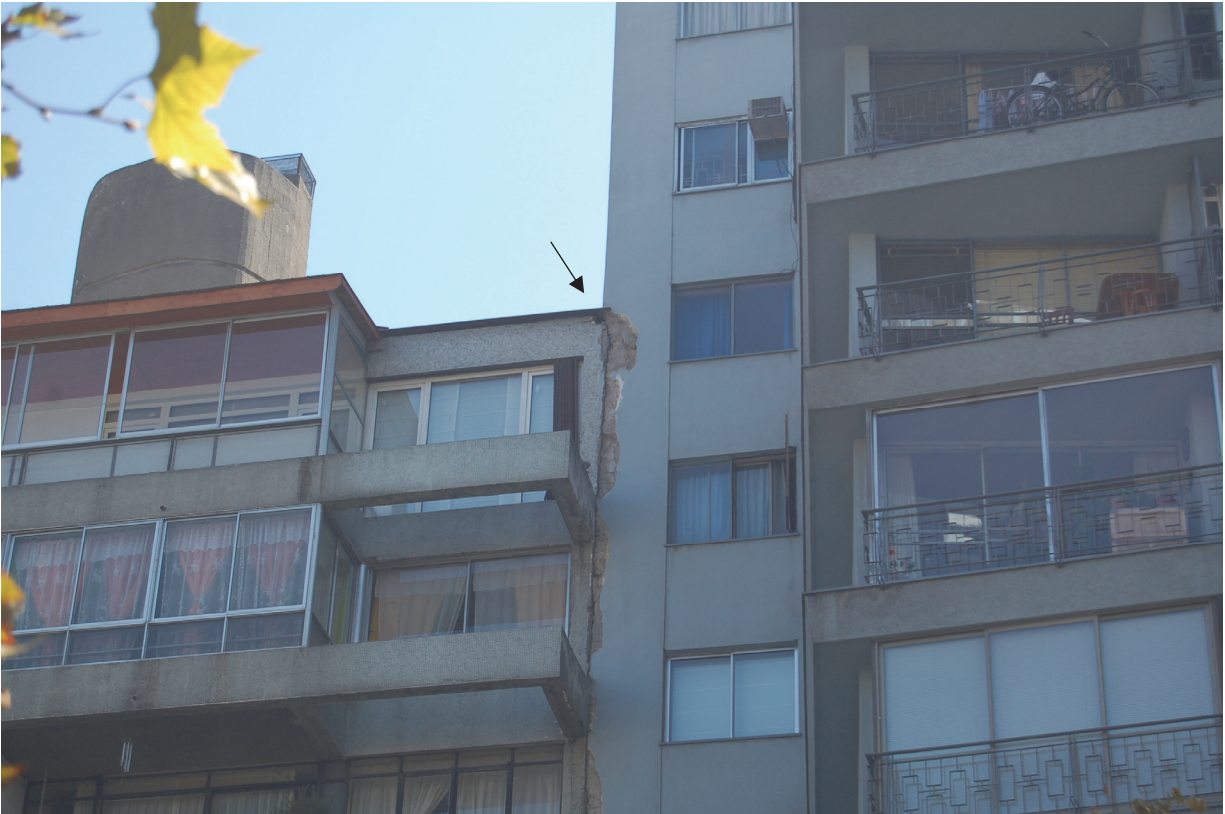
Figure 4-15 Pounding damage on two buildings in Santiago, Chile, following the 2010 Chile Earthquake.
