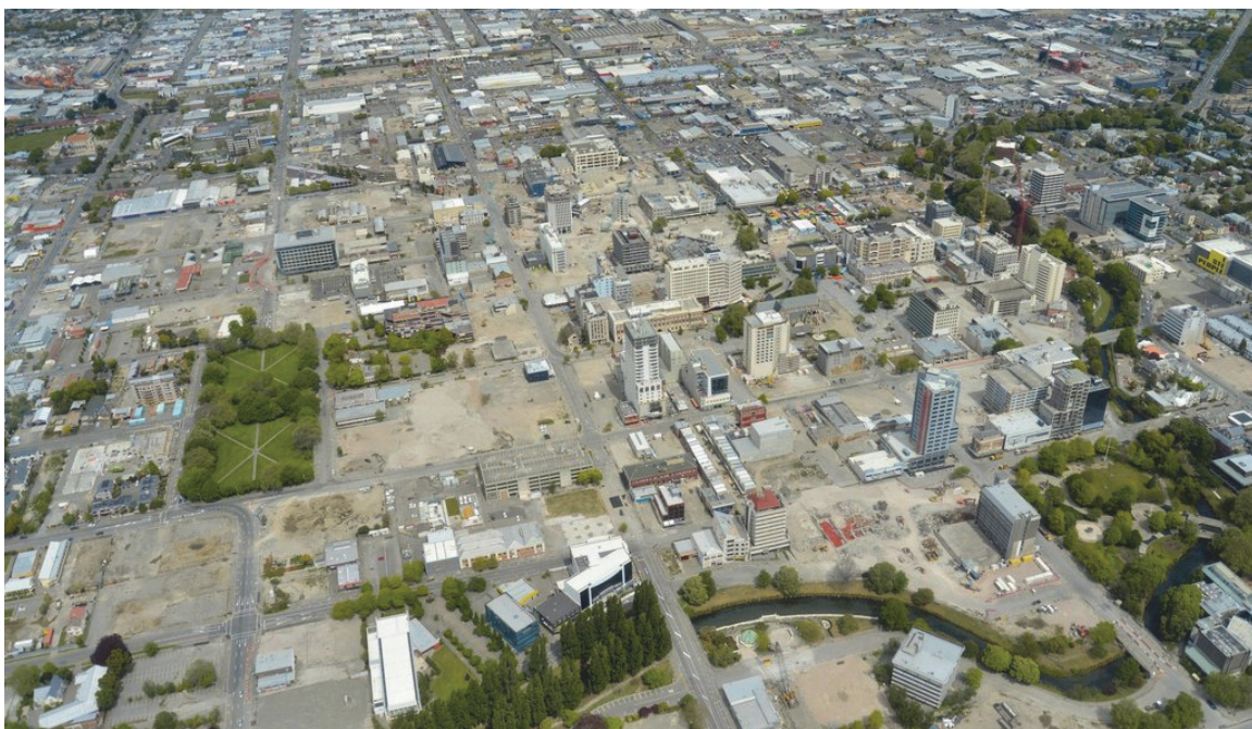
Figure 3-2 Christchurch, New Zealand after demolition of many buildings in the Central Business District following the 2011 Christchurch Earthquake (from Miyamoto International).
