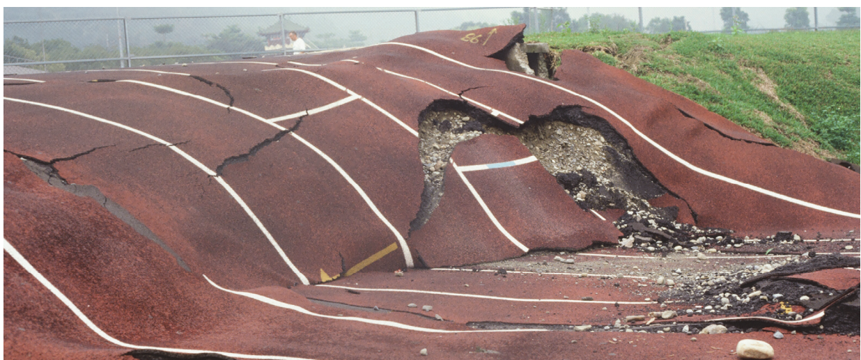
Figure 1-15 Vertical fault offset of a school track from surface fault rupture in the 1999 M7.7 Chi-Chi Earthquake in Taiwan (from B. Yeats).
