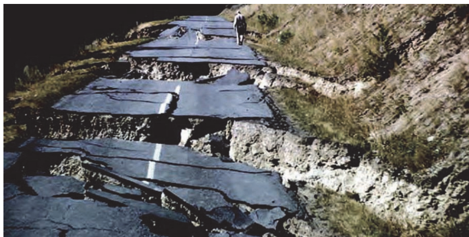
Figure 1-12 Lateral spreading damage to a highway in the 1959 Hegben Lake Earthquake (from USGS).
