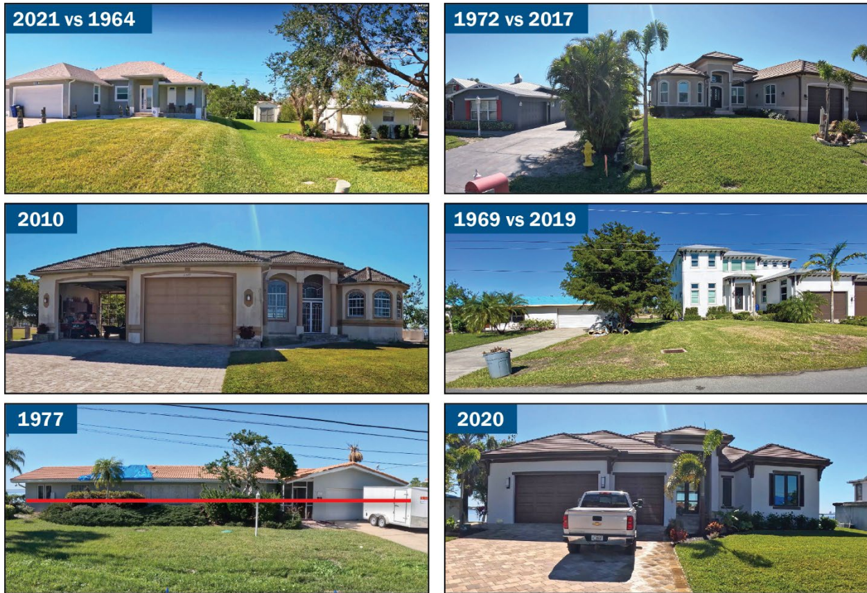
Figure 6: Representative single-family houses in Area of Interest No. 2 from the 1960s to 2020
