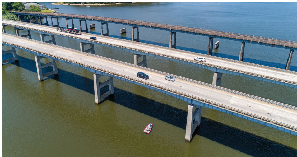
Photo Source: South Carolina Department of Transportation
