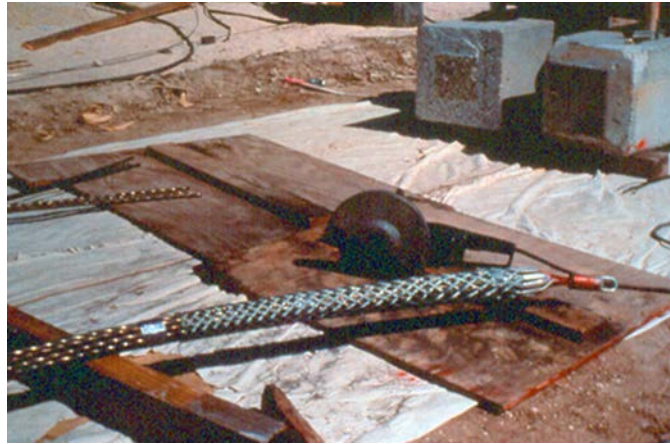
Figure 1.24– Bundled Tendon Prepared for Pulling
