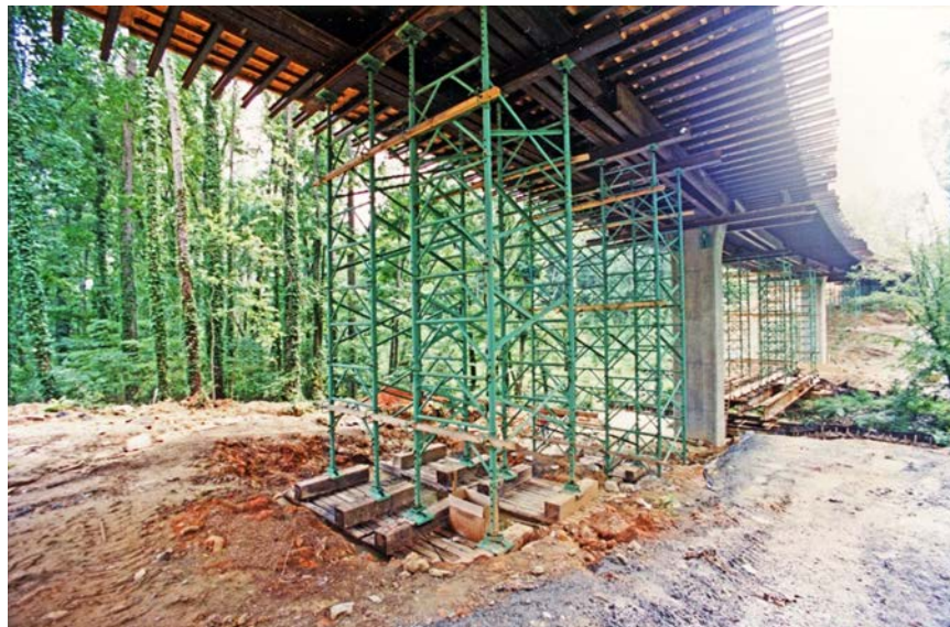
Figure 1.17 – Modular Falsework Units for Cast-in-Place Construction
