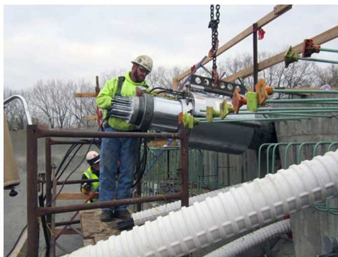
Figure 1.25– Stressing Post-Tensioning Tendons
