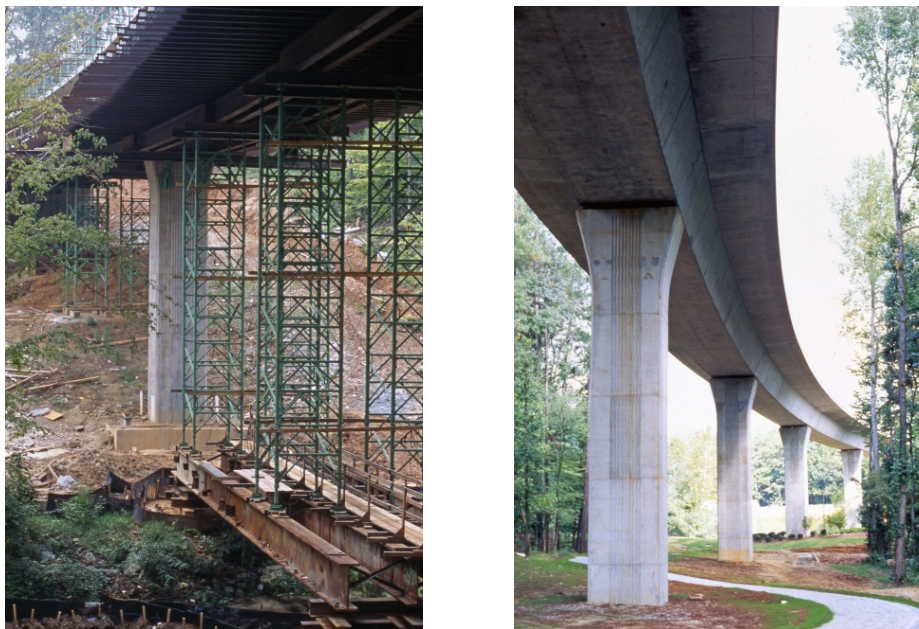
Figure 1.1 – Cast-in-Place Post-Tensioned Box Girder Bridge for the Metropolitan Atlanta Regional Transit Agency (MARTA) – under construction (left), completed (right)
