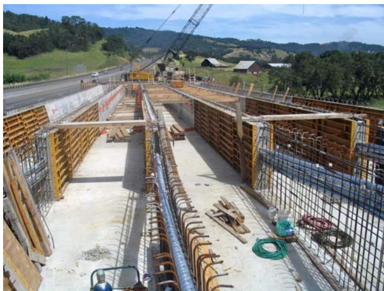
Figure 1.20 – Web Formwork for a Multi-Cell Box Girder
