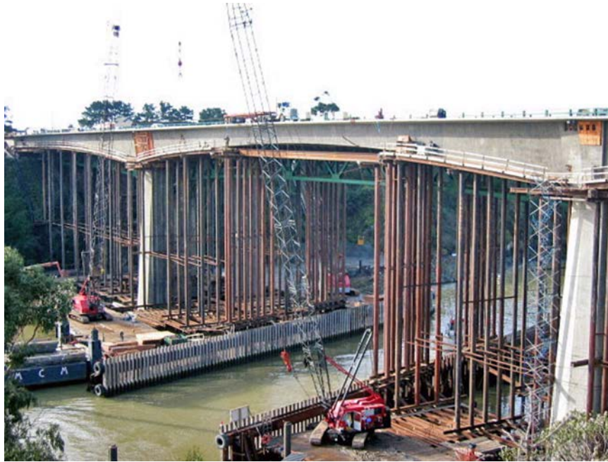
Figure 1.18 – Steel Pipe Support Towers for Cast-In-Place Construction
