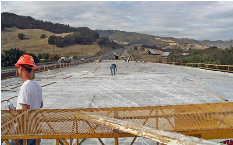
Figure 1.23– Curing the Concrete Deck
