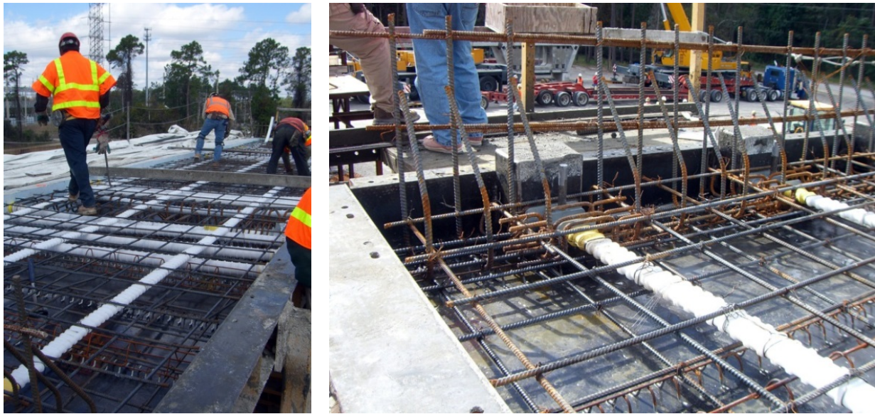
Figure 8.37 – Transverse Duct Placement in Casting Machine
