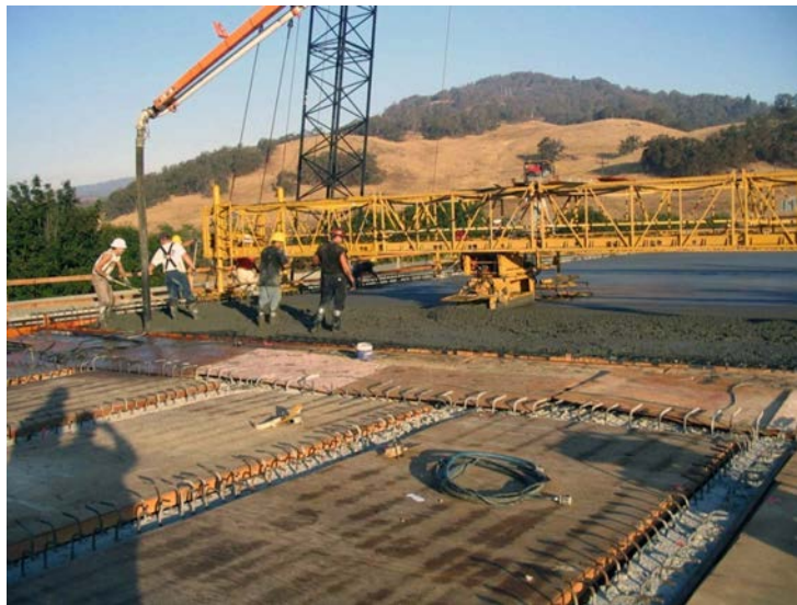
Figure 1.22 – Placing Deck Concrete and Finishing with a Roller Screed
