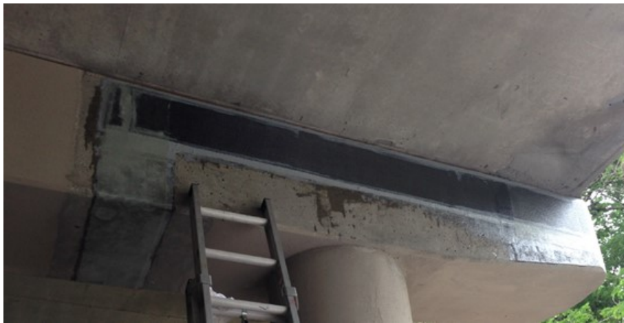
Figure 9. Photograph showing an externally bonded FRP repair.
