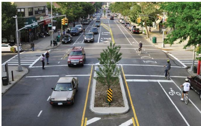
Figure B.6: Roadway Island Barrier
