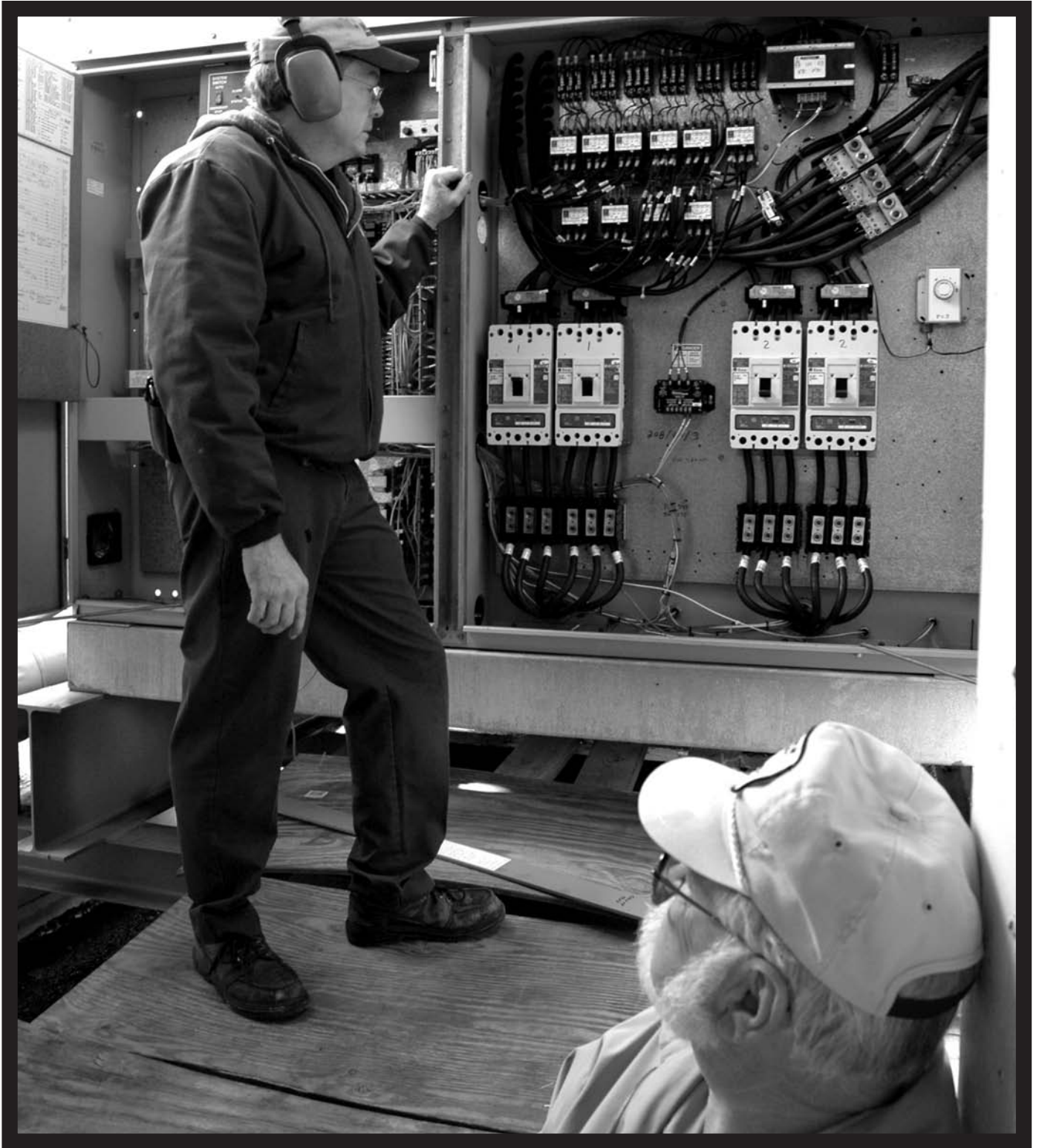
Maintenance technician Patrick Glennon (left) and Pete Gailey are seen here working on the air conditioning unit at Mount Carmel Gardens. Rehab, repairs and an upgrade to the air conditioning unit were completed using EHCL and HOME funds.
