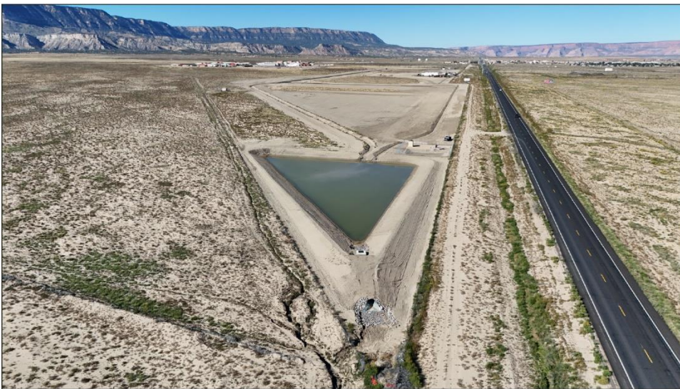
Figure 9: Abandoned Mine Land Economic Revitalization Project at Kayenta Industrial Park in the Navajo Nation
