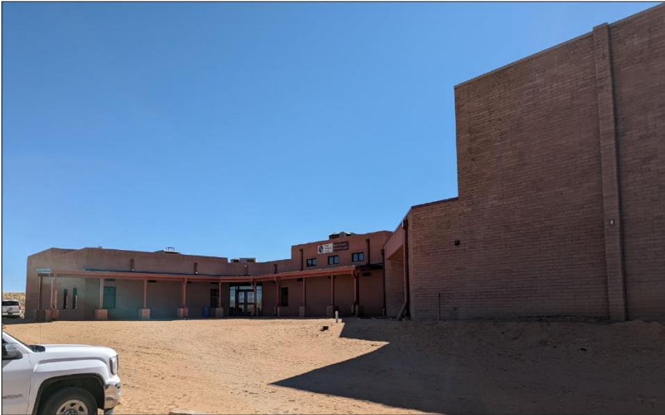
Figure 12: Hopi Wellness Center and Hopi Veterans Memorial Center Expansion Near Kykotsmovi Village, Arizona, Which Is Expected to Receive Abandoned Mine Land Economic Revitalization Program Funding
