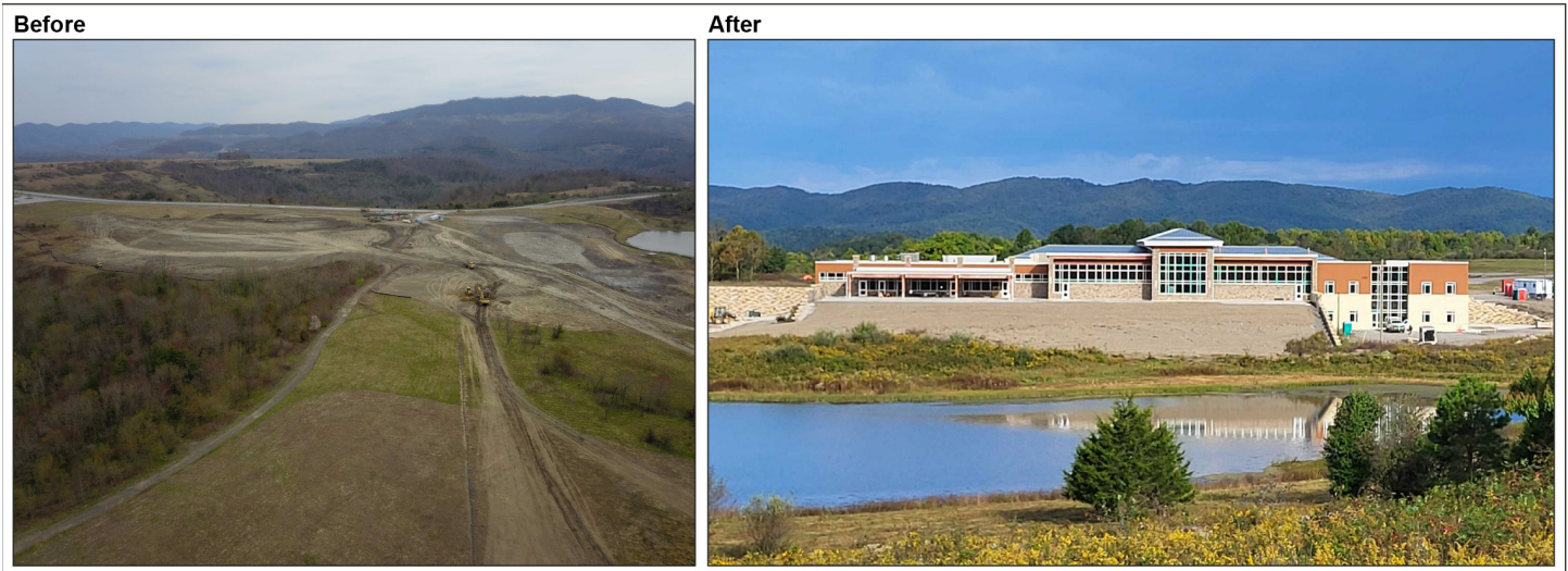
Figure 6: Appalachian Wildlife Center (Boone’s Ridge) in Kentucky, before and after Receiving Abandoned Mine Land Economic Revitalization Program Funding
