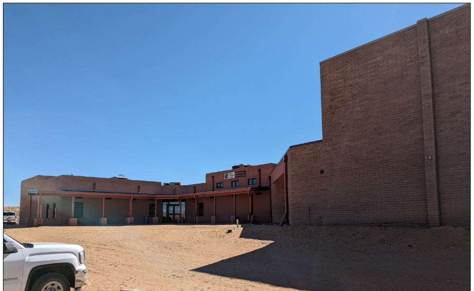
Figure 12: Hopi Wellness Center and Hopi Veterans Memorial Center Expansion Near Kykotsmovi Village, Arizona, Which Is Expected to Receive Abandoned Mine Land Economic Revitalization Program Funding
