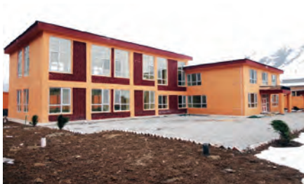
Provincial council administrative building completed under GPI in Panjshir Province, August 2017. (MCN Photo)
