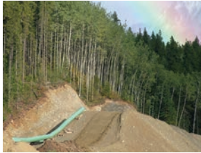
Welded sections of a pipeline Photo: Canada Energy Regulator
