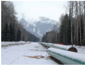
A pipeline being prepared for underground installation Photo: Canada Energy Regulator
