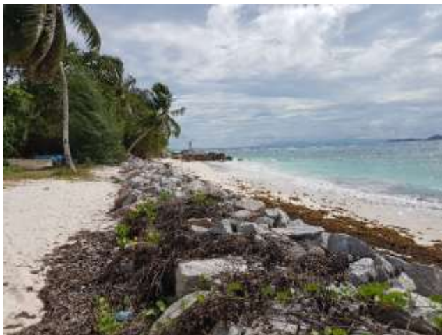
Picture 17: Coastal Degradation and Rock armouring being used at Anse Kerlan Beach
