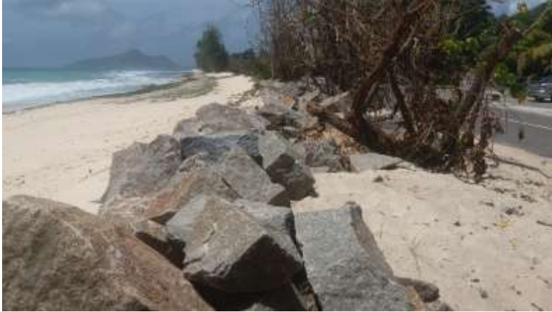
Picture 19: Rock Dumping at North East Point
