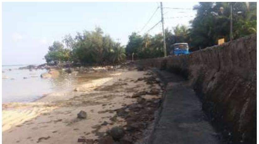
Picture 2: The above road at low tide showing the concrete revetment used
