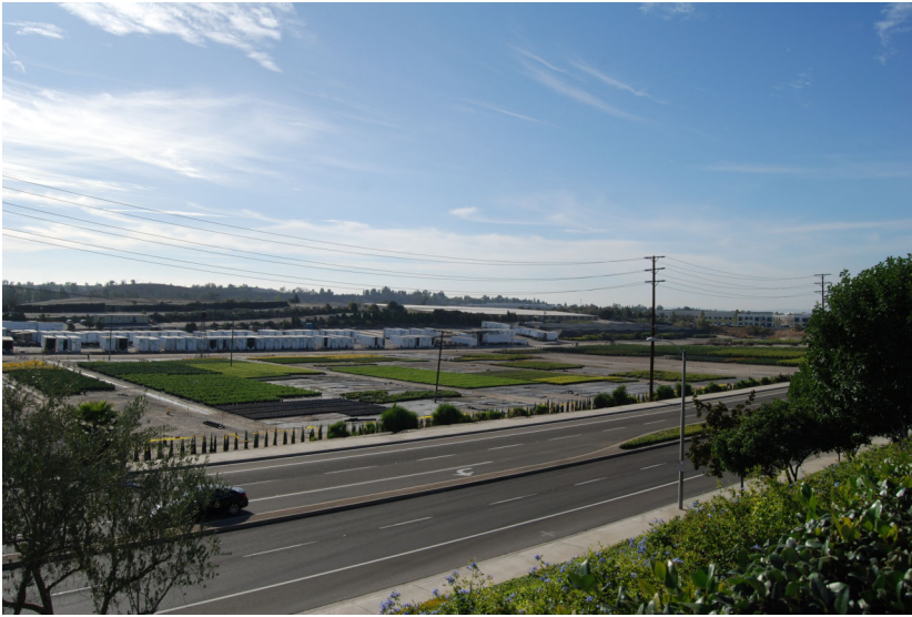
View facing south from Bake Parkway.
