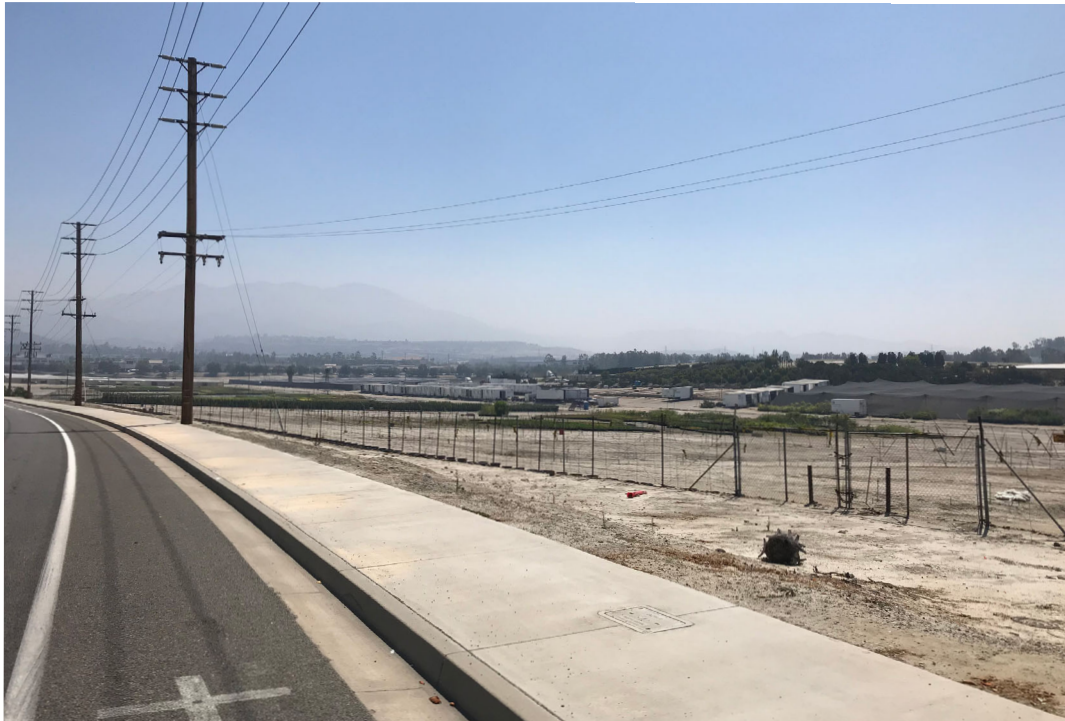
Existing Condition - View from Bake Parkway looking northeast.
