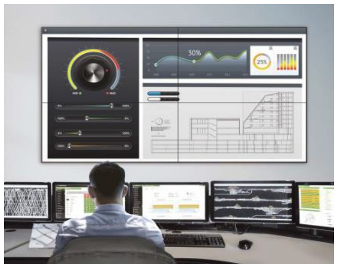
Figure 12 Small control room
