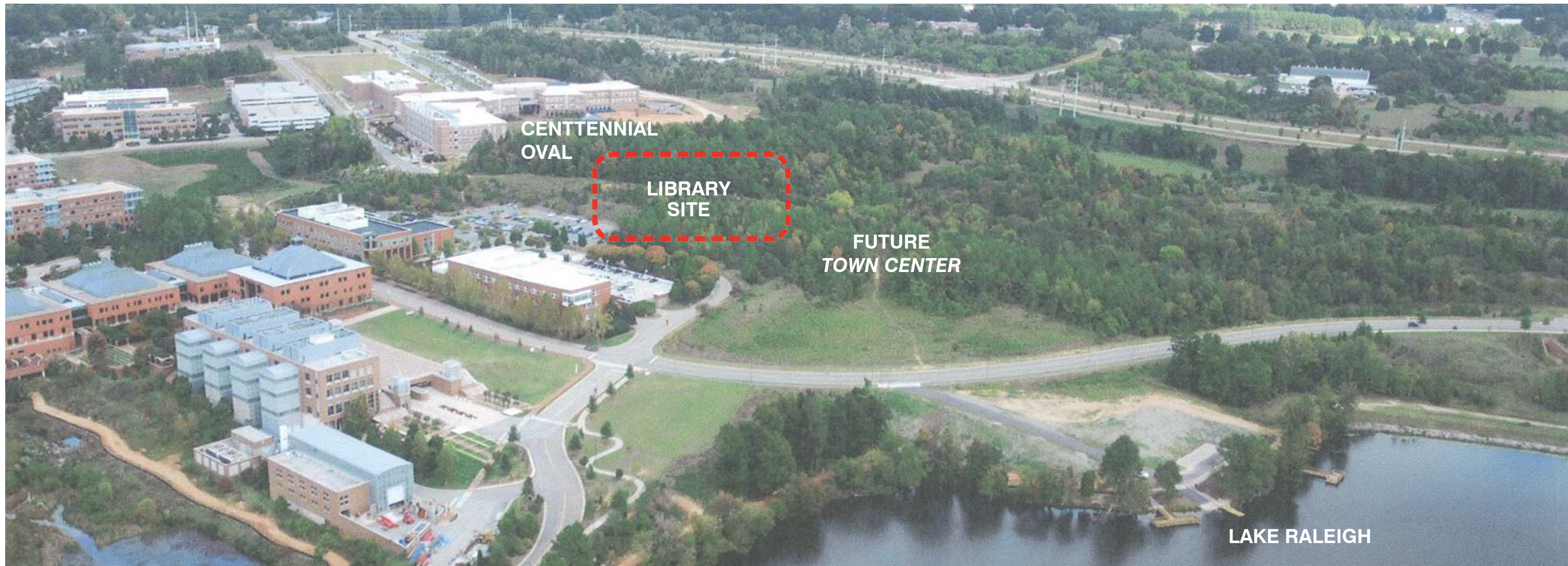
Aerial Image - Centennial Campus
