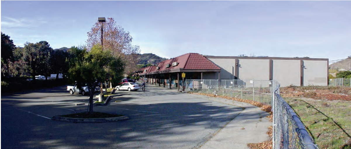
Existing shopping center.
