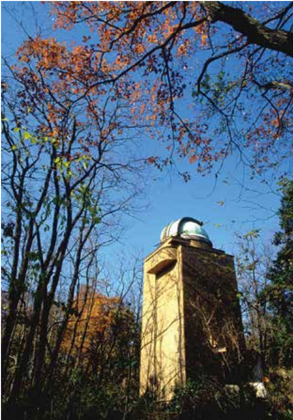
▲Solar Tower Telescope (Einstein Tower) at Mitaka Campus. It became a registered tangible cultural property in 1998.
