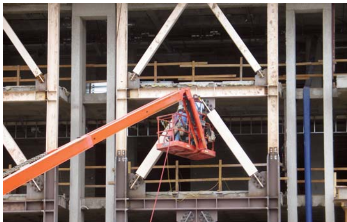
Unbonded steel braces are used as part of the seismic rehabilitation of the J. Willard Marriott Library on the University of Utah campus. FEMA provided partial funding of this project through the PDM grant program (Photo credit: Kelly Peterson, University of Utah).
