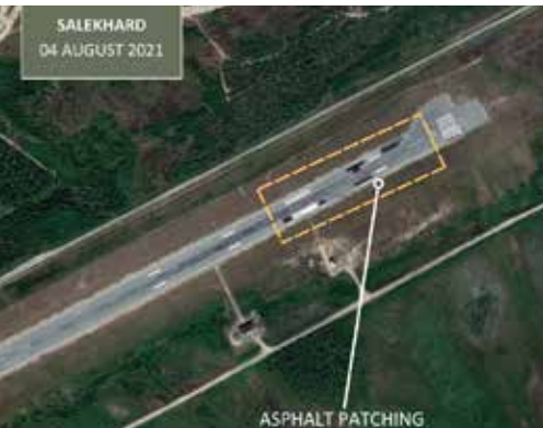
Figure 67: Patchwork repairs at Salekhard 2021 Google Earth 08/04/2021
