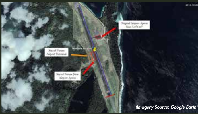
Figure 8: Imagery from December 2012 illustrates the location of the original airport apron prior to the renovations and the sites of the future airport terminal and apron. The original size of the apron was 5,476 m 2 .
