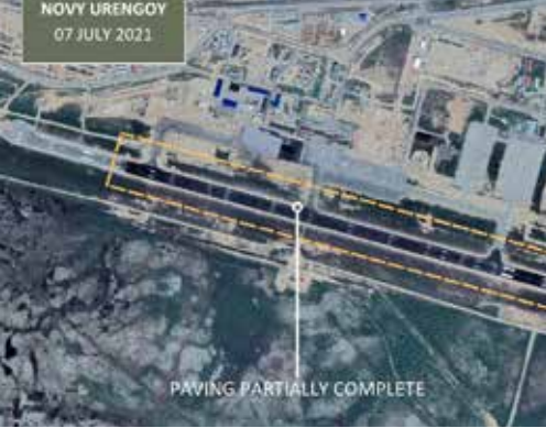
Figure 63: Paving at Novy Urengoy Google Earth 07/07/2021
