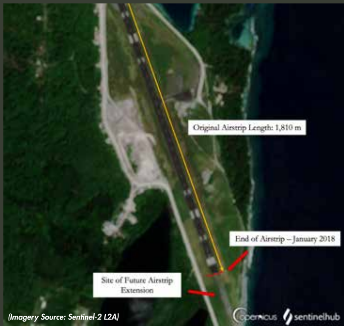
Figure 3: The Momote Airport's airstrip measured 1,810 meters in length on January 7, 2018.
