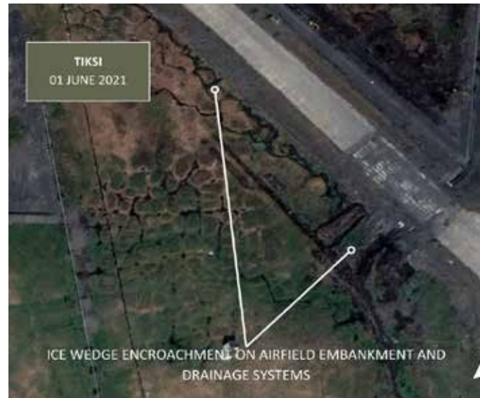
Figure 92: Ice wedges south of the runway Google Earth 06/01/2021
