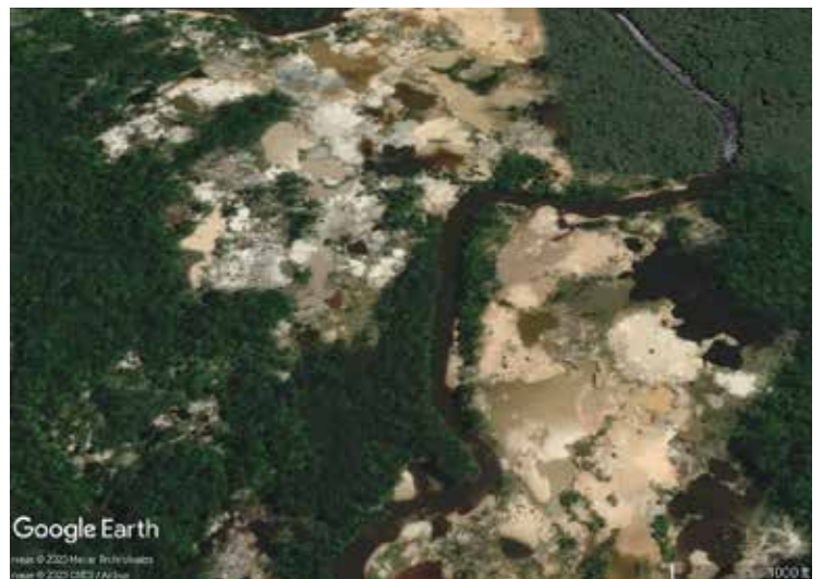
Figure 15: Image showing spoon-like holes and ponds with brownish water at Mining Site 13 Google Earth Pro, 5/23/2020
