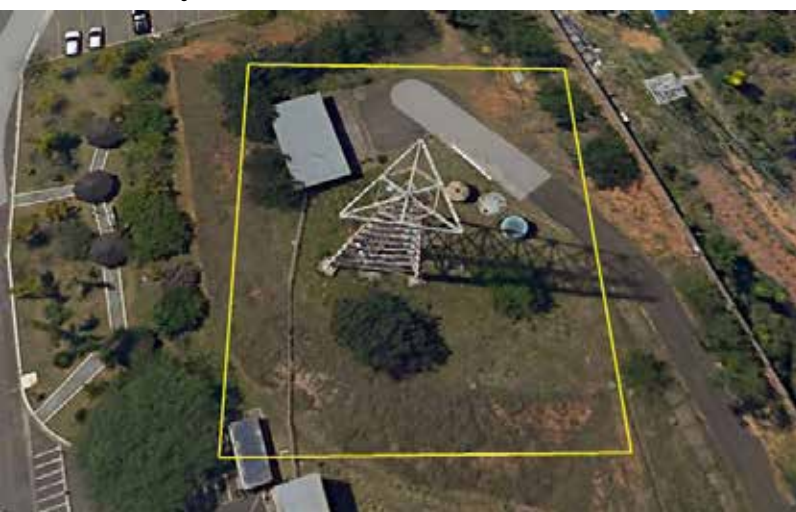
Figure 6: Possible Cell Tower (Zoomed view). Source: Google Earth November 2022
