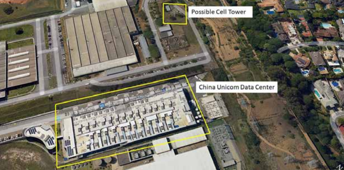
Figure 5: China Unicom Data Center in São Paulo, Brazil. Source: Google Earth November 2022
