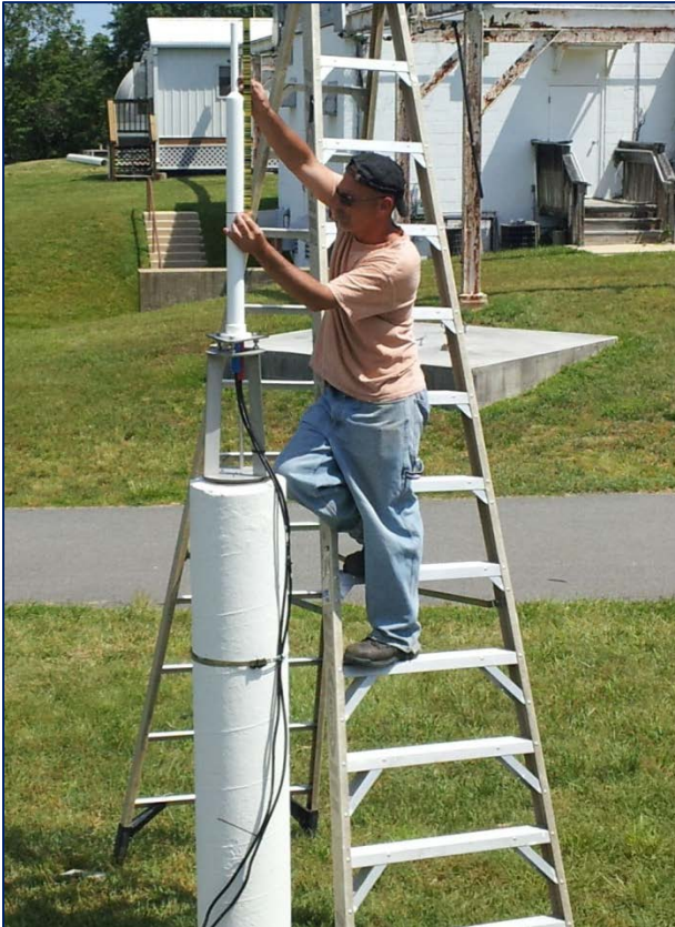
Figure 17. Carefully leveling to the DORIS ARP, the midpoint of a red band encircling the tube.
