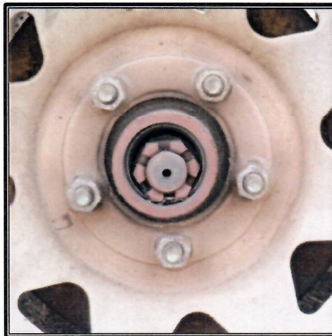
Right-Rear Spindle with Missing Dust Cap
