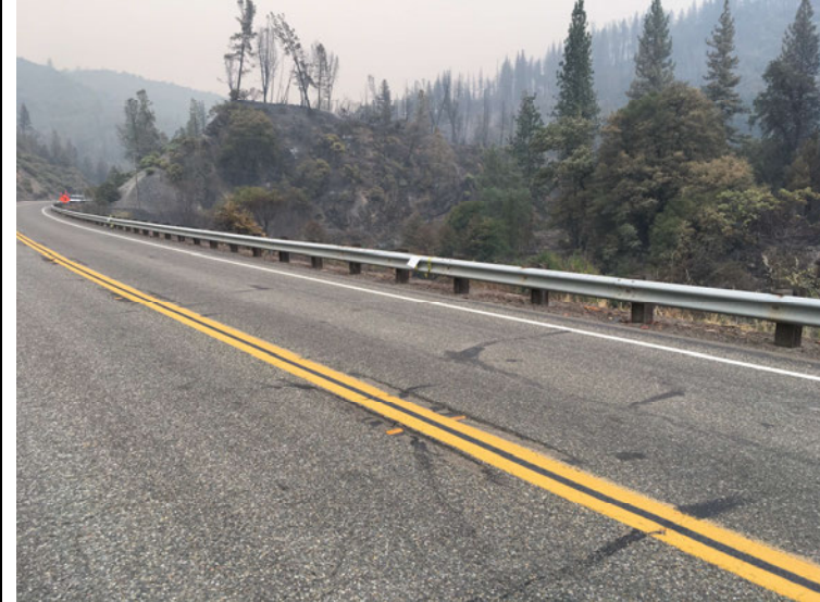
Photo Number: IMG_0797 Photographer: U.S. Park Ranger N. HENKE, Badge Number 1024 Date and Time: 07-31-2018 / 1701 hours Subject: CARR FIRE – photos of the origin areas along the highway (near mile marker 9) – flagging and signage added to preserved guardrail areas until further assessment can be completed by (b) (7)(C), (b) (6) – looking approximately Southeast
