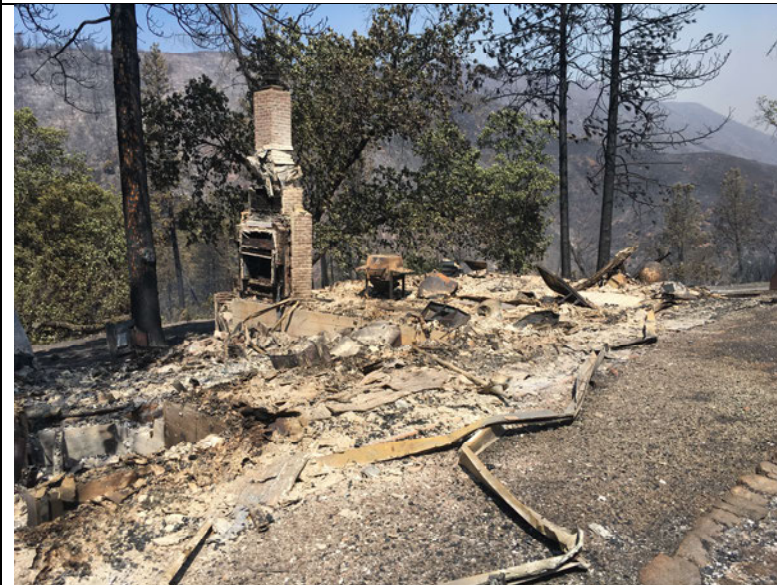
Photo Number: IMG_0782 Photographer: U.S. Park Ranger N. HENKE, Badge Number 1024 Date and Time: 07-24-2018 / 1104 hours Subject: CARR FIRE – Quarters 515 – another view of residence
