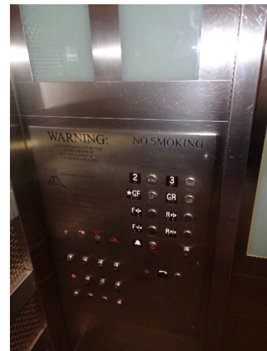
4. Existing car station is to be replaced.
