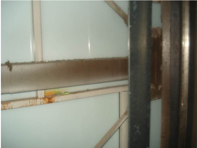
5. Clean down hoistway
