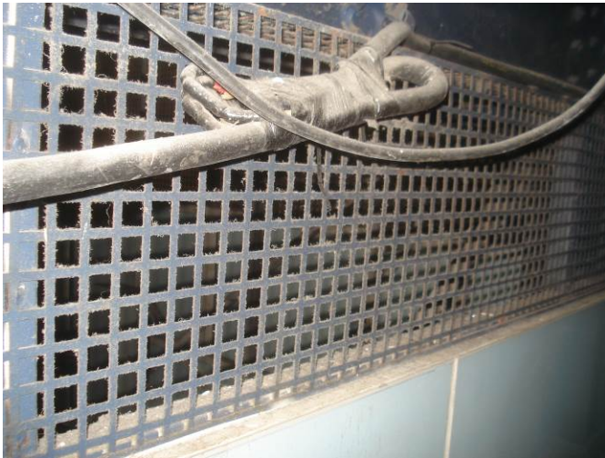
21. Clean hoistway outside of dust, dirt and debris
