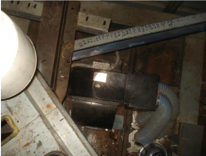
13. Replace electrical cover on cartop fan and clean cartop
