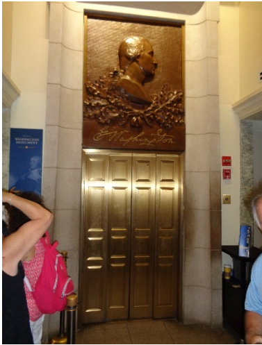
1. Existing lobby entrance doors to be retained.
