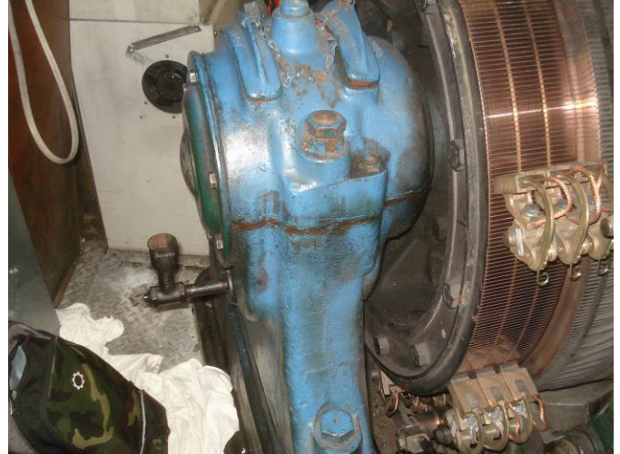
2. Clean hoist machine of accumulation of dirt
