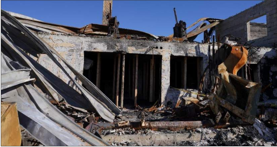
Figure 14 - South side of the concrete structure (looking north, August 17, 2023, TJB).
