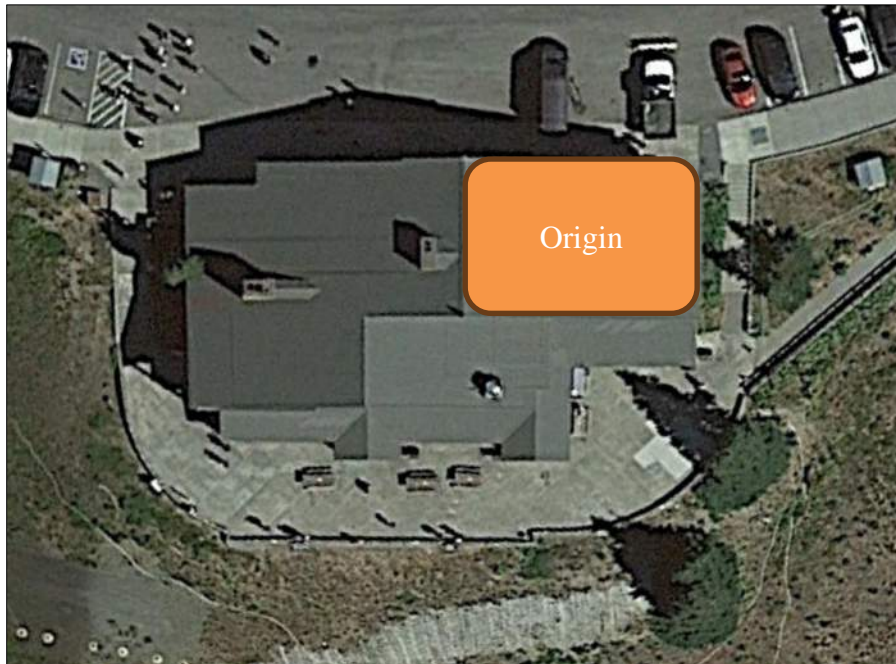
Figure 1 – Area of Fire Origin – Pre-fire image.
