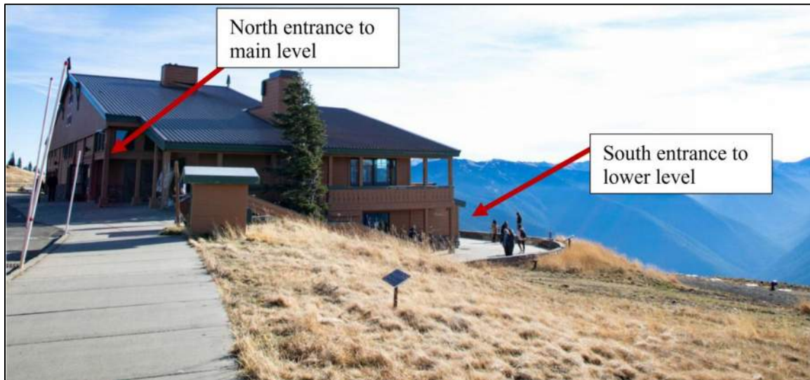
Figure 2 - HRDL Construction - Entrances
