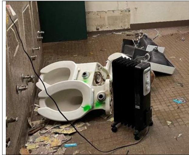
Figure 5 - Radiant Heaters utilized at HRDL. (April 19, 2023)
