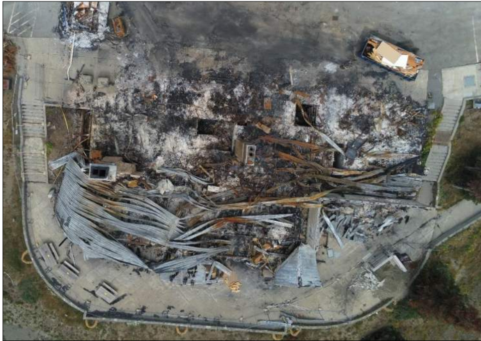
Figure 20 – NPS Drone Image - August 22, 2023.
