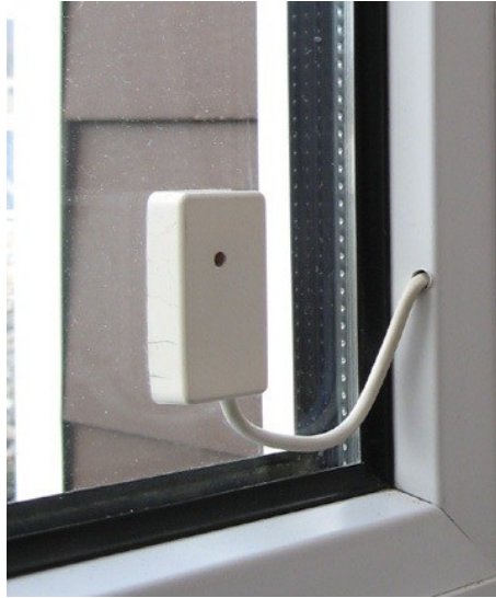
Figure 4-6 Glass-break sensor
