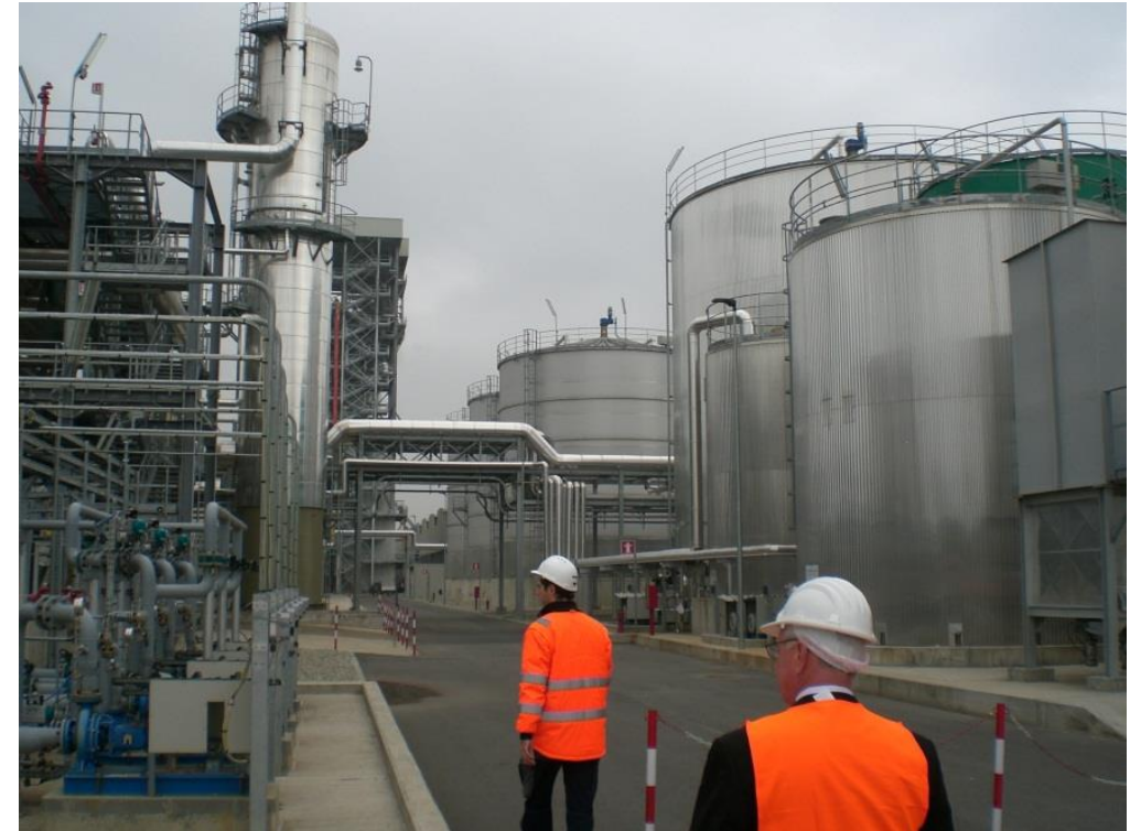
Cellulosic biorefinery, Crescentino, Italy.
