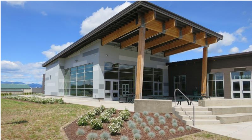
New Bridge High School
