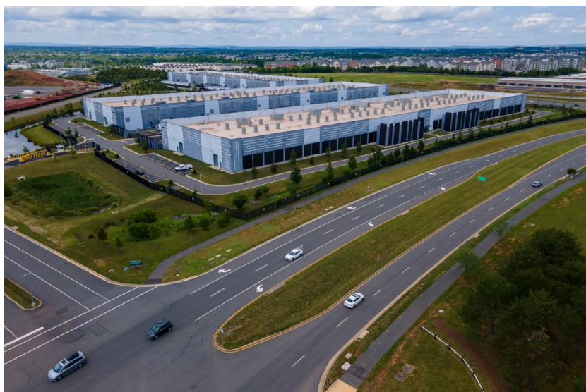
Data centers in Ashburn, in Loudoun County, Virginia, house computer servers and hardware required to support modern internet use. Ted Shaffrey/AP Photo
