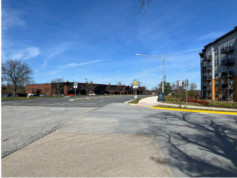
Photograph # 25 – Residential development (right) and office building (left) adjacent to study area along Annapolis Way (3/1/2024)
