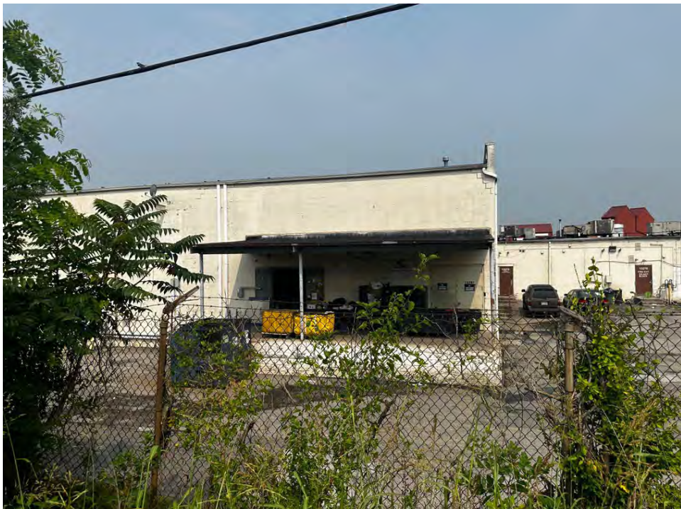
Photograph # 8 - Loading dock on east side of commercial buildings (7/13/2023)
