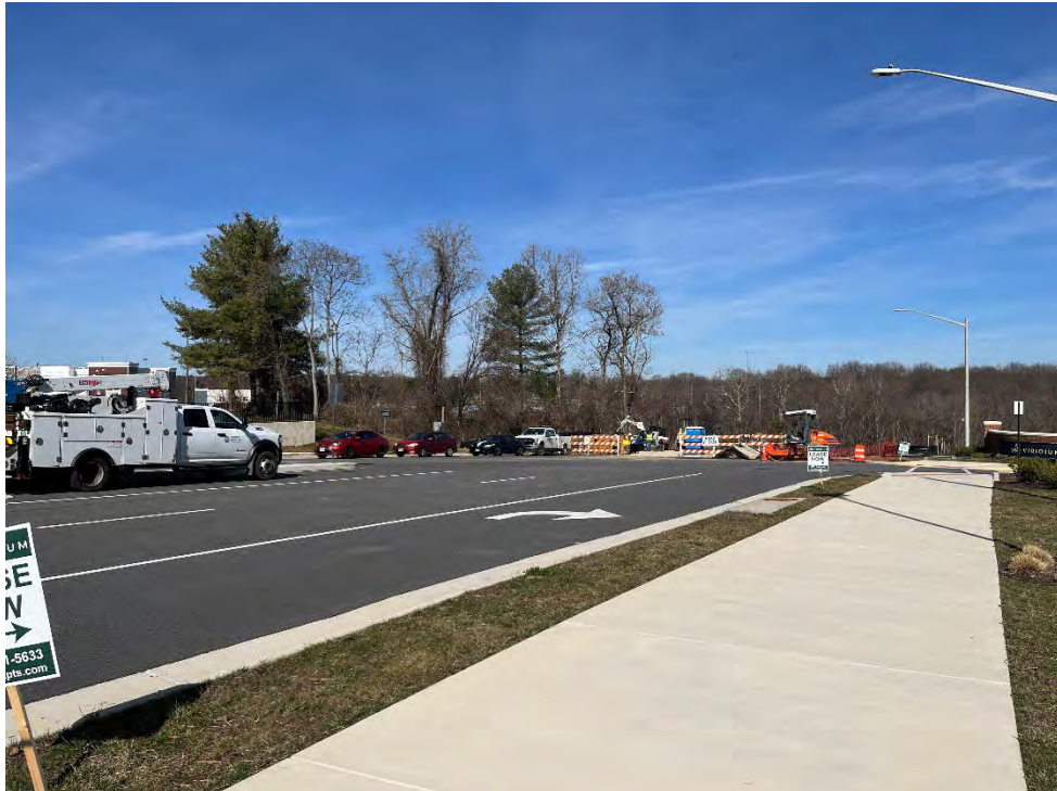
Photograph # 24 – Active roadway construction occurring immediately northwest of study area at existing terminus of Annapolis Way (3/1/2024)
