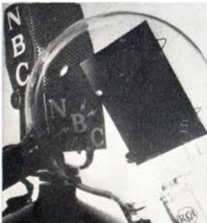
The Iconoscope, “eye” of the television camera.
