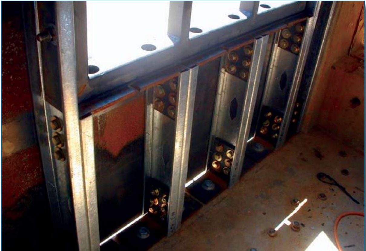
Figure 2-19 Metal stud blast wall
