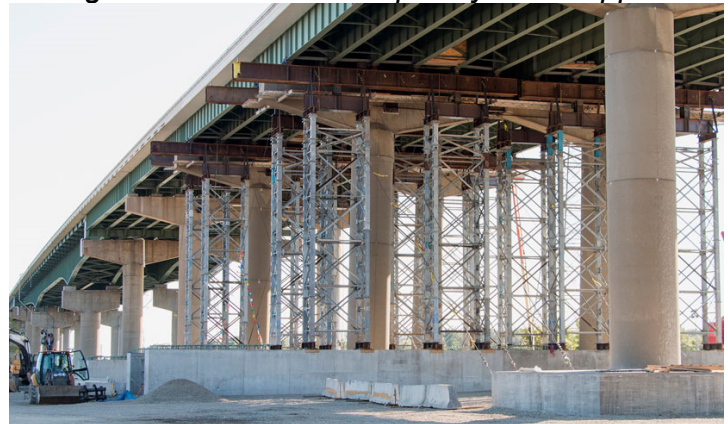
Figure C3 – EFCO Temporary Pier Support
