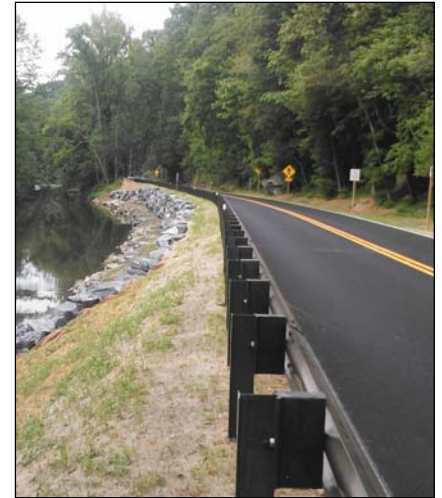
Corman Construction was the contractor for MSHA's first CMAR - MD 24 – Deer Creek Project
