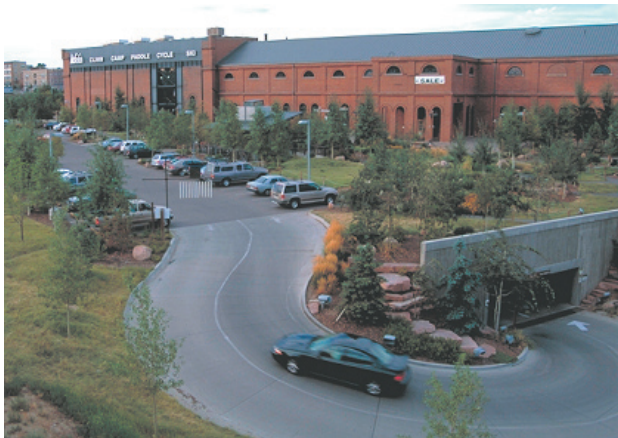
Underground and terraced parking structures can offer usable pedestrian space on their rooftops.
