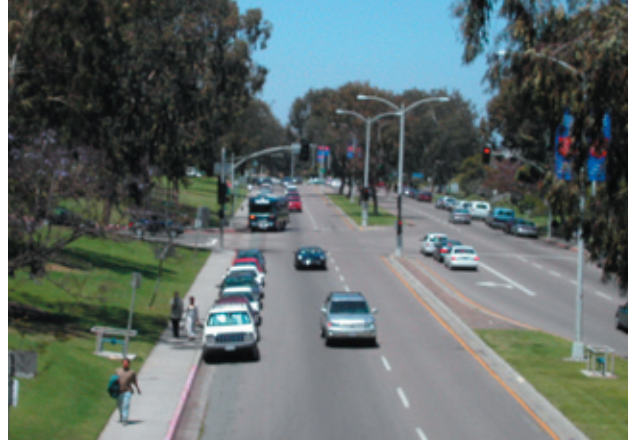
Attached walkways create an urban feel.
