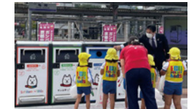
IoT-enabled garbage cans installed at Kameoka Station
