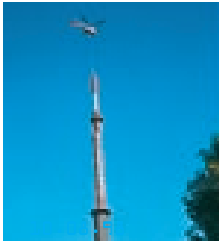
Interference-free, top-quality reception guaranteed: The new antenna is in operation.
