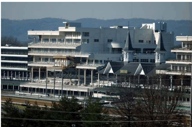
Churchill's 2001-2005 $121 million renovation was one of many improvements under the Meeker era. Horsephotos
