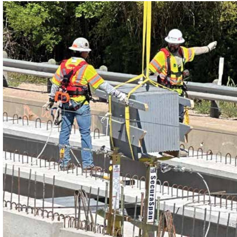
I-35 Capital Express North crews install new bat boxes under the rebuilt Walnut Creek frontage road. Photo by Jessica Duverney
