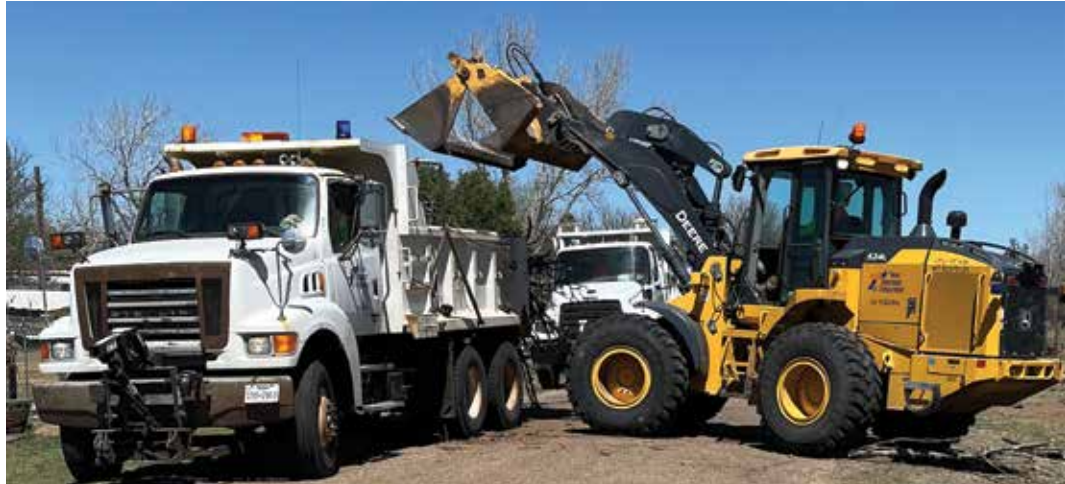
Amarillo District crews help with debris cleanup in the town of Fritch after devastating wildfires in February and March. Photo provided by the Amarillo District
