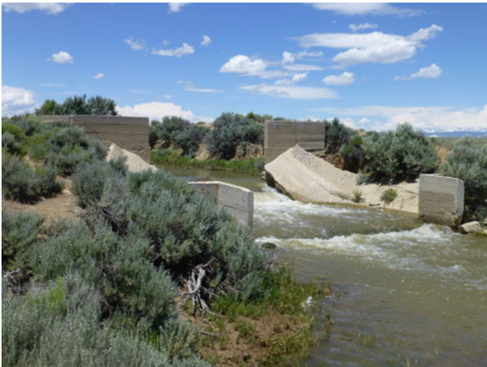
Figure D-4. Downstream side of the drop structure nearest to the headworks of the Big Sandy Feeder Canal.
