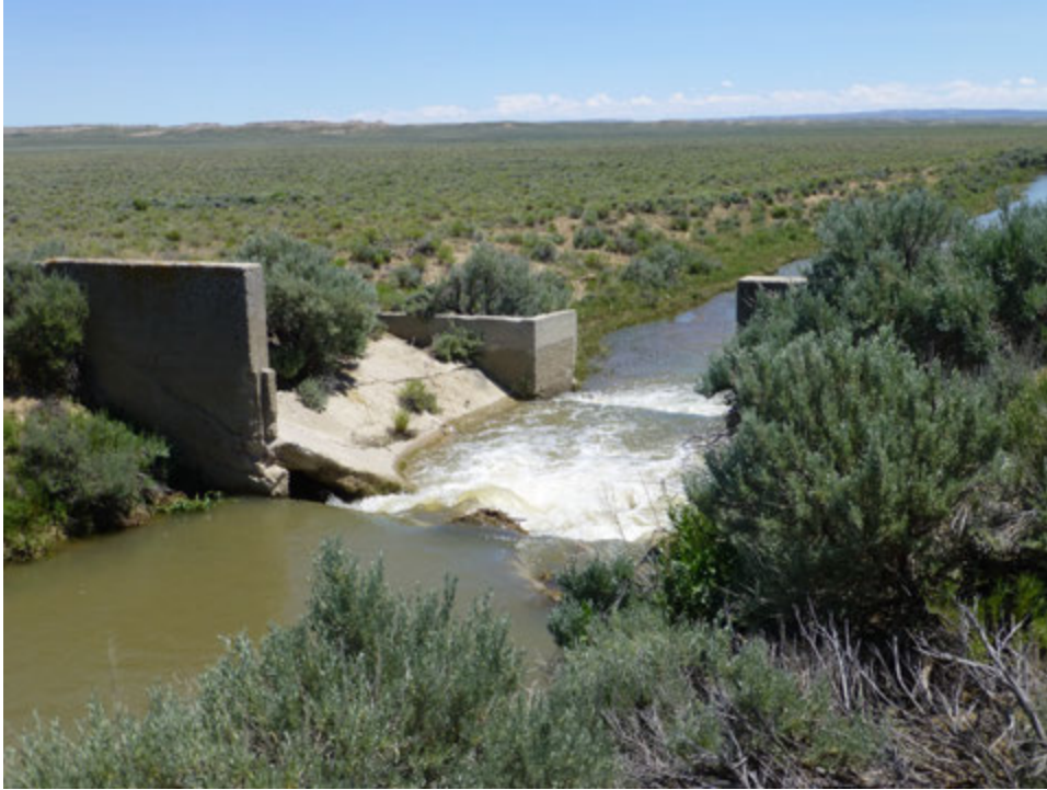
Figure D-3. Upstream side of the drop structure nearest to the headworks of the Big Sandy Feeder Canal.
