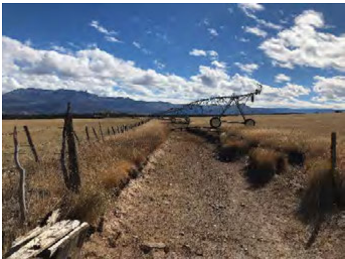
Gould Canal section 3, proposed for lining.
