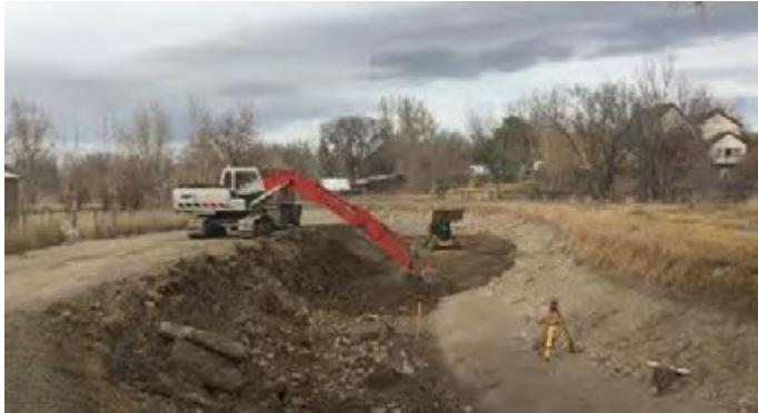
Example of canal preparation for lining.
