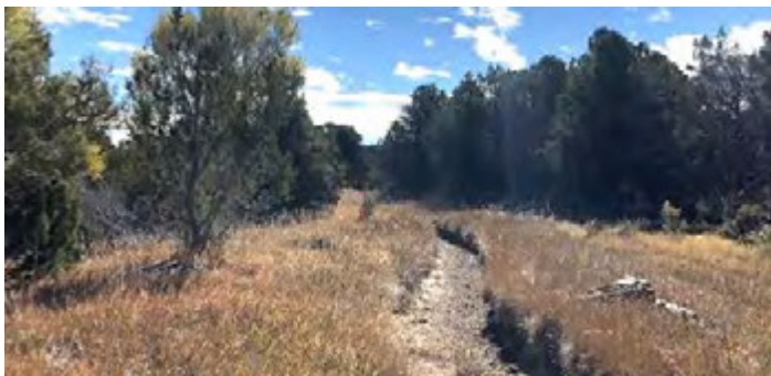
Gould Canal section 5, proposed for lining.
