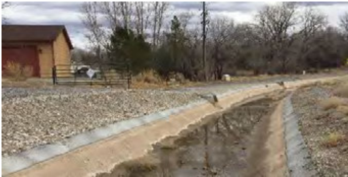
Example of a lined canal.
