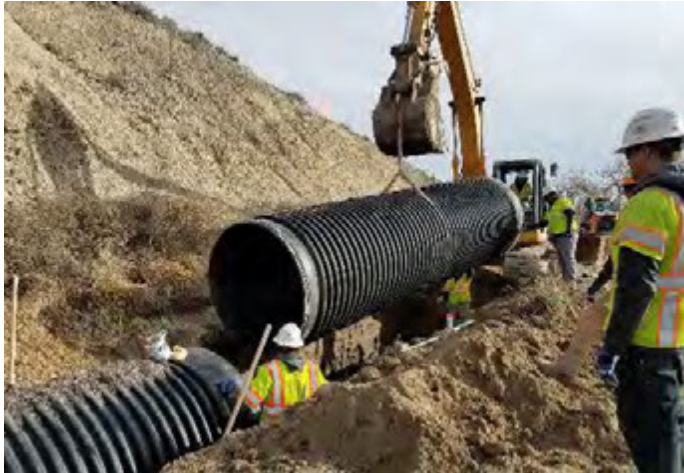
Example of pipe installation in an existing canal.
