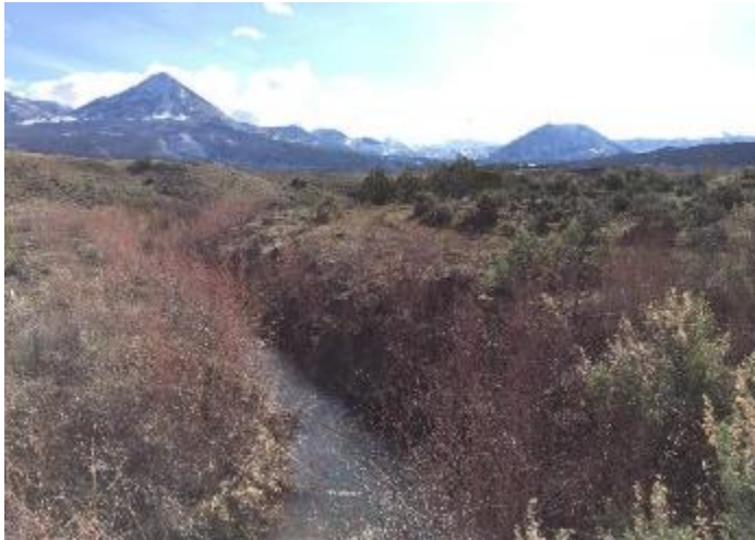
Photograph 1. Looking east along the Center Lateral on BLM land in the middle part of the Proposed Action Area.
