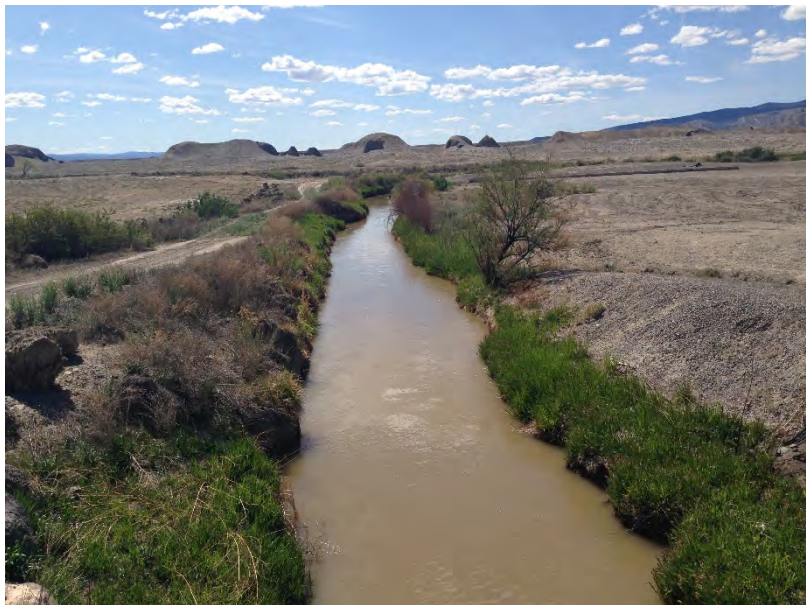
Photograph 2. West Project Area: typical appearance of the part of the canal that would be decommissioned and backfilled.
