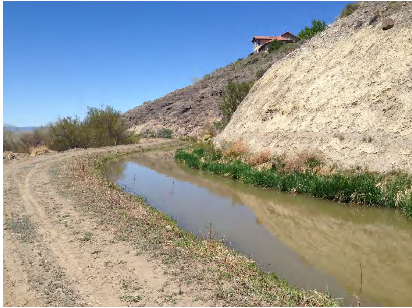
Photograph 1. East Project Area: typical appearance of the canal where the pipeline would be installed in the canal alignment.
