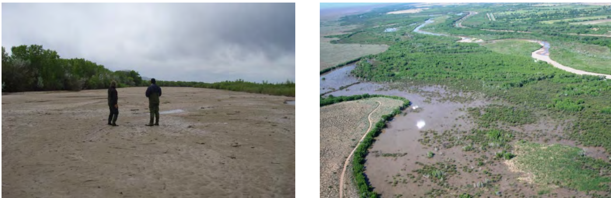
Figure 16 Sediment plug photos from 2008 (a) May 23, 2008: main channel is filled with sediment and all flow is forced around the plug into the floodplain (b) July 4, 2008: flows have receded and a large volume of water remains ponded in floodplain which will be the location of the new realigned channel .
